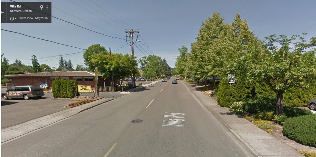
Figure 3 – Villa Road near HWY 99 – Looking North
