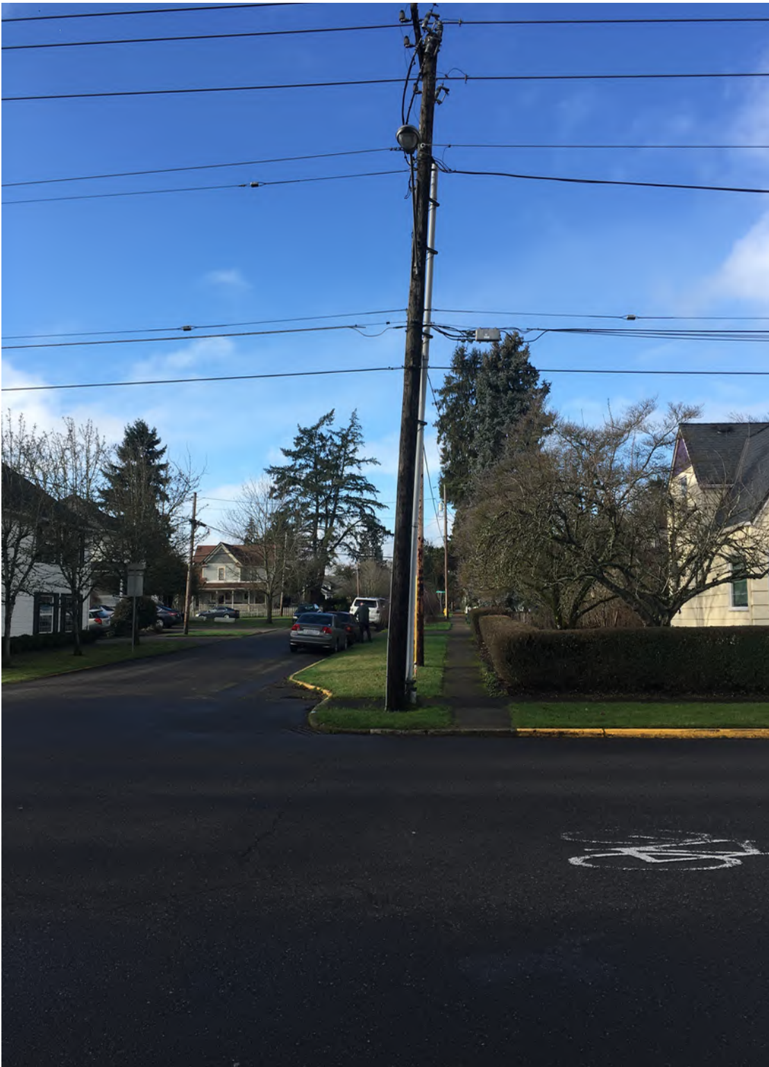
N Meridian Street/E Sheridan Street looking to the west from the northeast quadrant; Illumination is provided only on the northeast quadrant of the intersection
