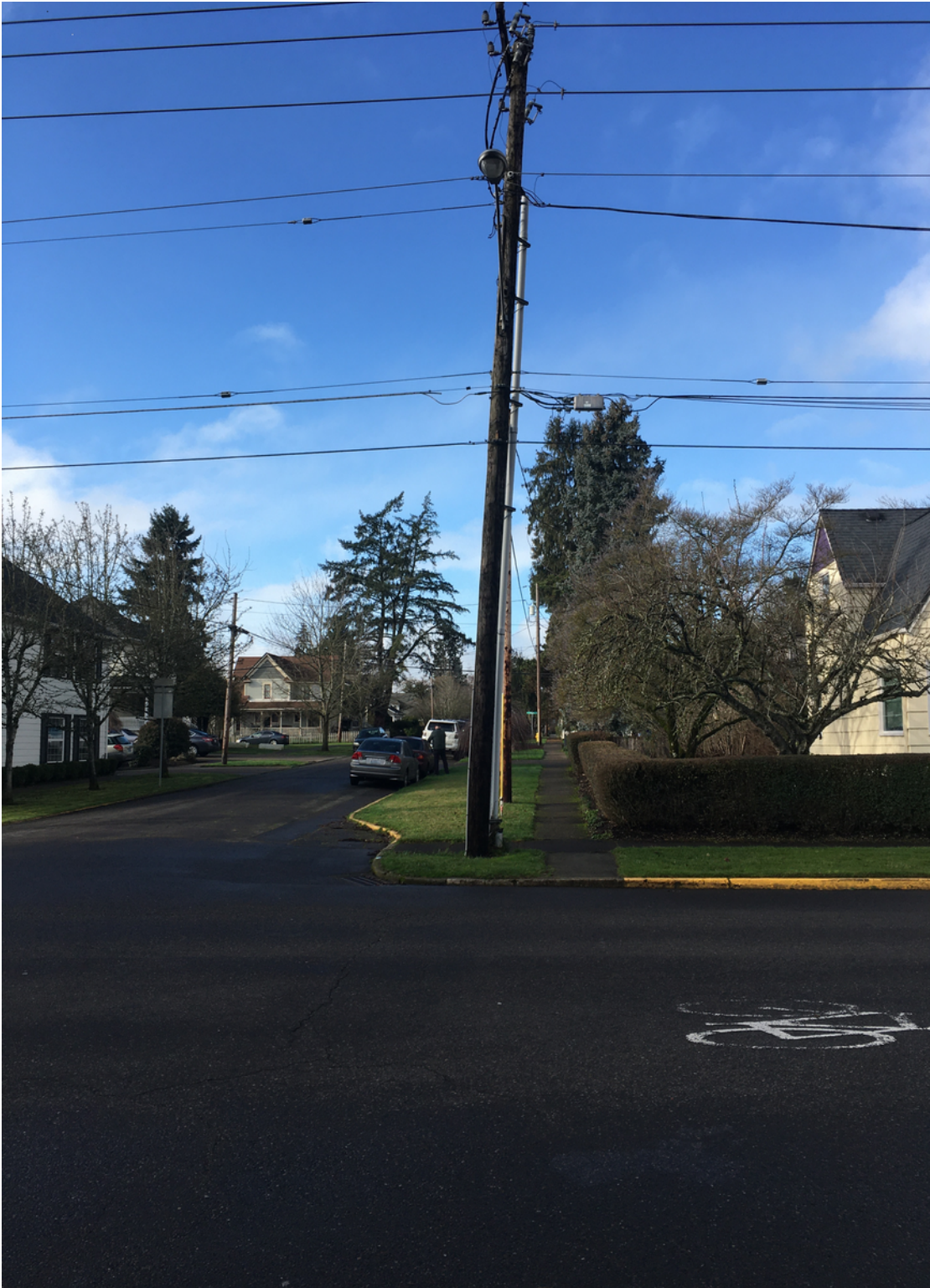
N Meridian Street/E Sheridan Street looking to the west from the northeast quadrant; Illumination is provided only on the northeast quadrant of the intersection
