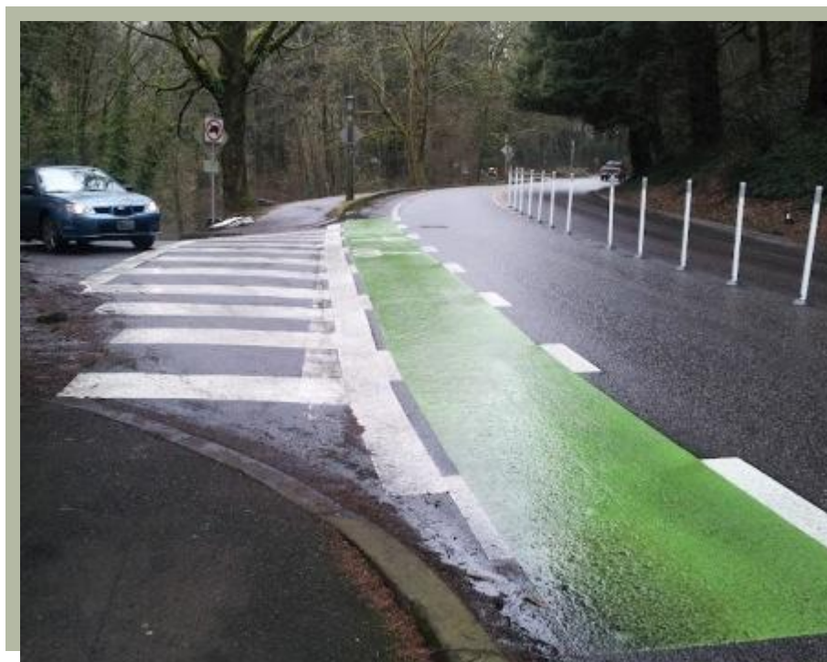
Figure 8: Example of Plastic Bollards along the Street Centerline restricting left-turns
