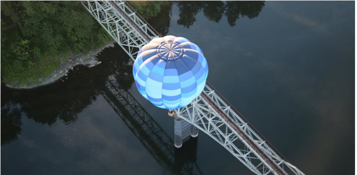
FIGURE 24. VIEW OF WATERLINE BRIDGE, A POTENTIAL LOCATION FOR A BICYCLE/PEDESTRIAN CROSSING OF THE WILLAMETTE
