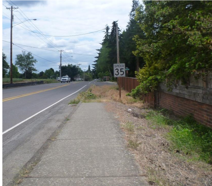
Gaps in Sidewalks on Arterial Roadway
