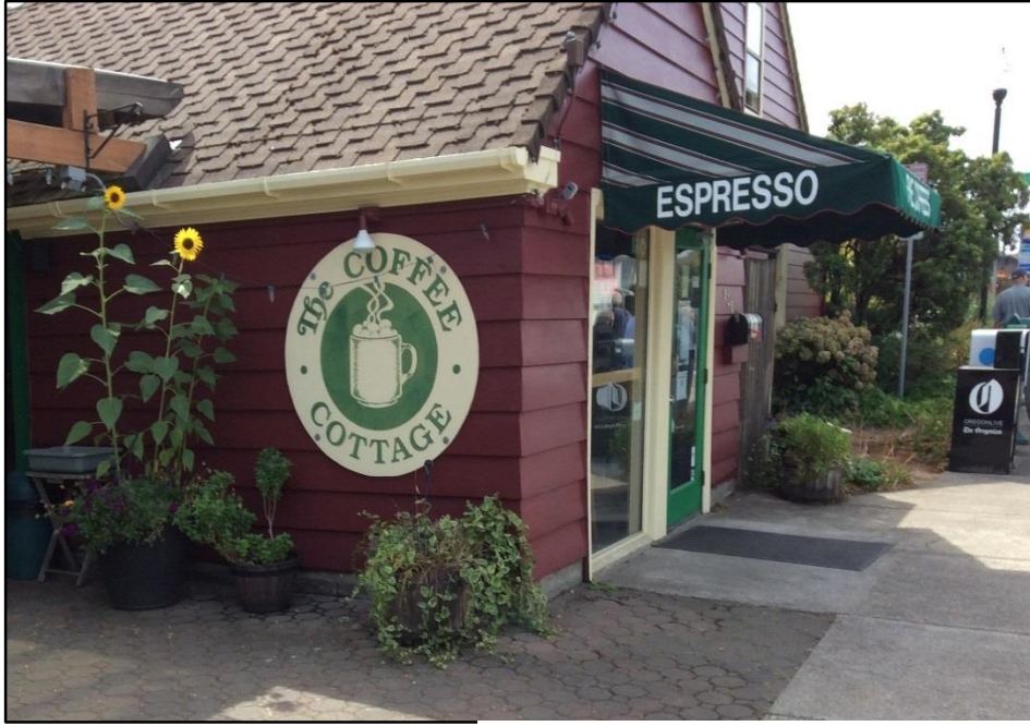
Photo 1. Re-Use building on Hancock Street.
