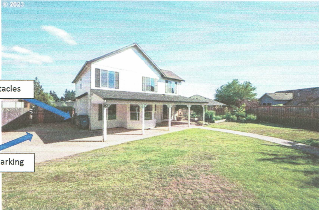
Exterior rear of House
