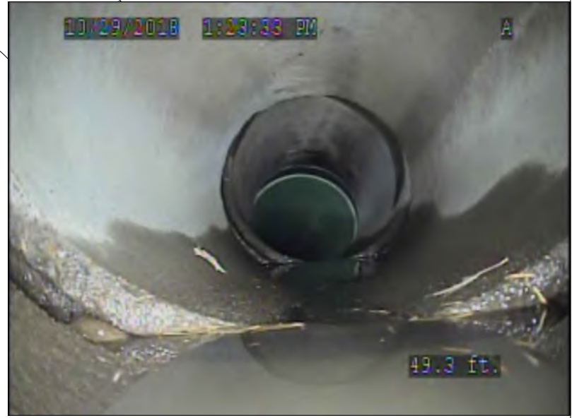
FIG. 1: SEPARATED JOINTS IN EX. STORM PIPE
