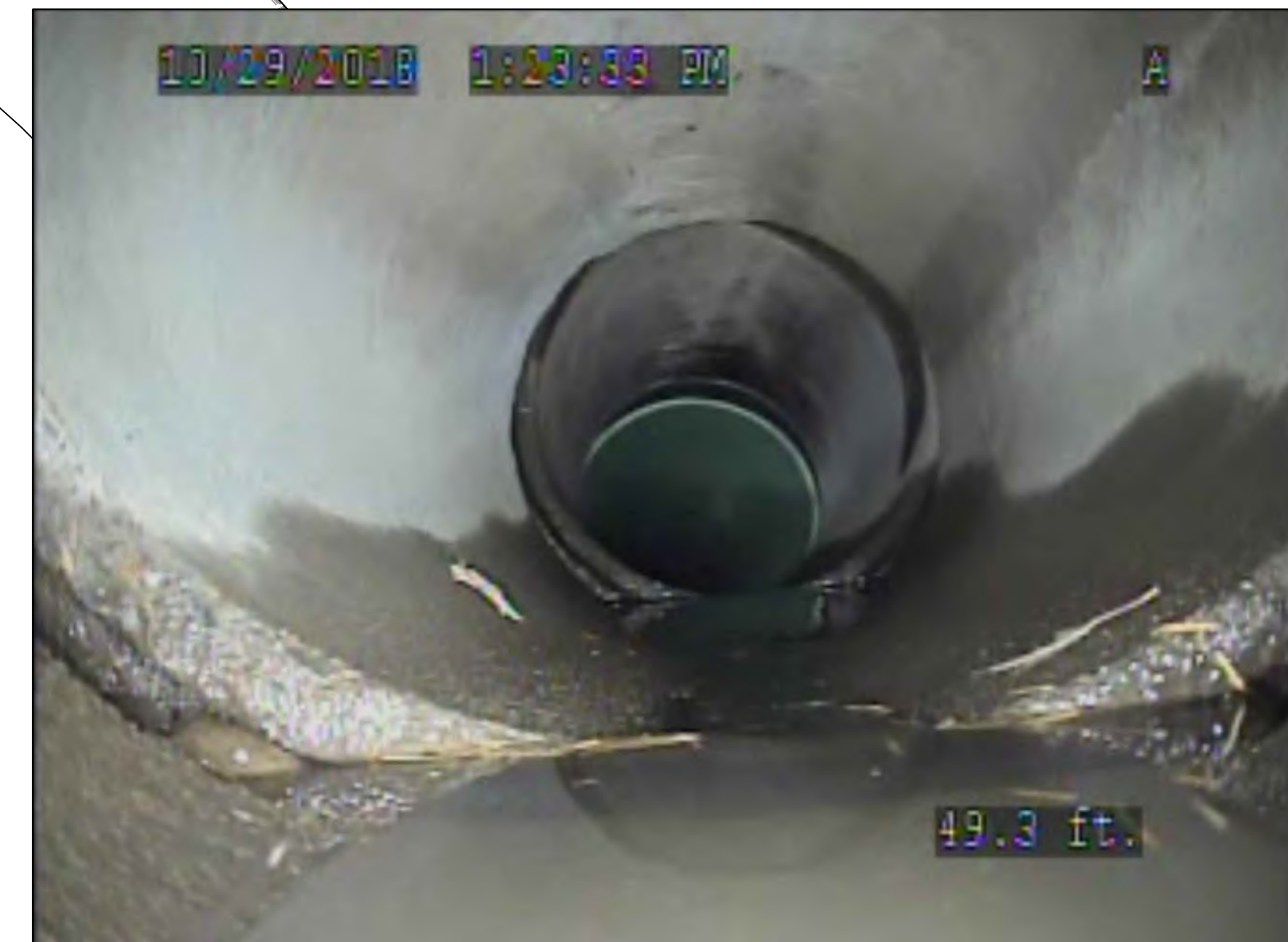
FIG. 1: SEPARATED JOINTS IN EX. STORM PIPE
