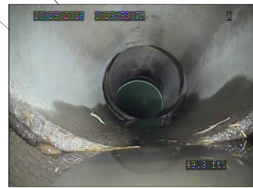
FIG. 1: SEPARATED JOINTS IN EX. STORM PIPE
