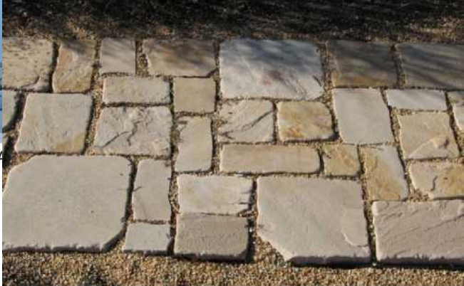
SEMI-PERMEABLE PAVER PATHWAY
