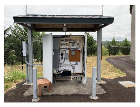
Figure 3.2 – Electrical Panelboard and SCADA Equipment Enclosure and Canopy
