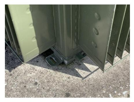
Figure 3.96 – Electrical Transformer not Anchored to Concrete Pad
