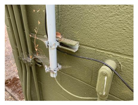
Figure 3.10 – SCADA Antenna Supported with Friction Clips
