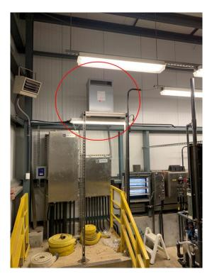
Figure 3.90 – Transformer not Adequately Braced
