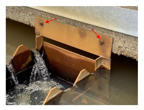
Figure 3.52 – Weir Trough to Basin Structure Connection Using Small Diameter Anchors
