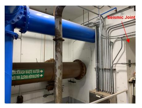
Figure 3.62 – Finished Water Sample Pipe and Filter Backwash Pipe Cross Seismic Joint without Adequate Flexibility
