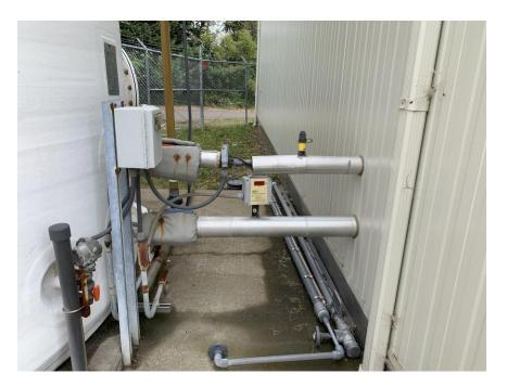
Figure 3.80 – Piping Connecting Salt Brine Tank to Sodium Hypochlorite Generation Building without Adequate Flexibility
