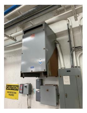
Figure 3.69 – Electrical Transformer not Adequately Braced Against Movement Parallel to Wall
