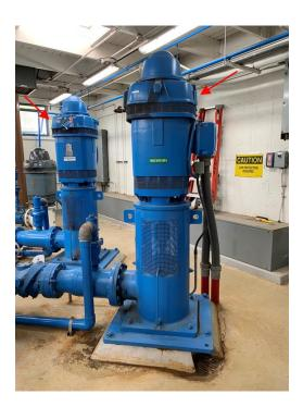
Figure 3.68 – Pump Motors not Braced to Structure Above their Center of Gravity
