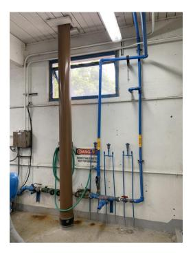
Figure 3.67 – Air Relief Piping Penetrating Laterally Unrestrained
