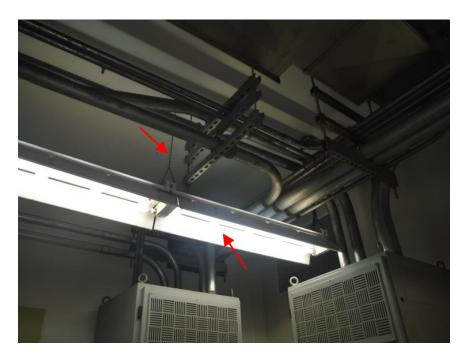
Figure 3.29 – Lights on Pendant Supports not Restrained and without Lens Covers
