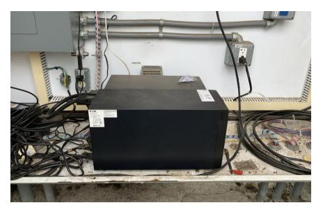
Figure 3.3 – Unrestrained Backup Batteries
