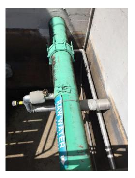
Figure 3.53 – Raw Water Pipes Penetrating Concrete Wall without Adequate Flexibility Through Wall
