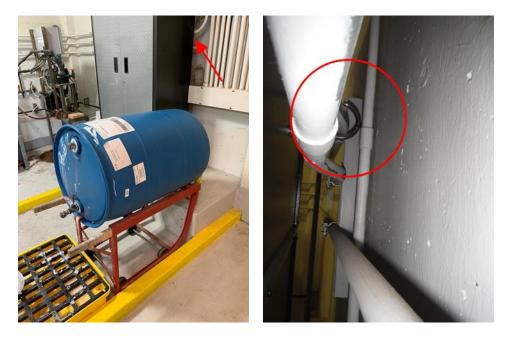
Figure 3.22 – Storage Cabinet Restrained with U-Bolt to Electrical Conduits
