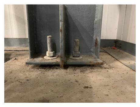
Figure 3.79 – Ungrouted Base Plate and Nuts on Anchor Rods not Tight
