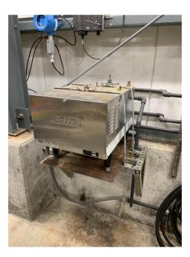
Figure 3.88 – Instant Hot Water Heater not Adequately Restrained
