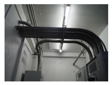
Figure 3.26 – Electrical Conduits not Seismically Braced and without Flexible Connections to Cabinets
