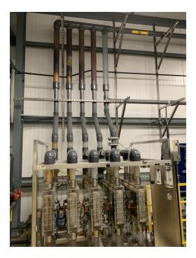
Figure 3.84 – Lack of Flexibility in Piping between Sodium Hypochlorite Generator and Attachment to Building
