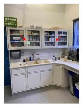
Figure 3.44 – Chemical Cabinet Doors without Proper Latches
