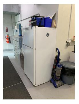
Figure 3.30 – Unrestrained Refrigerator and Filing Cabinets Adjacent to Walkway
