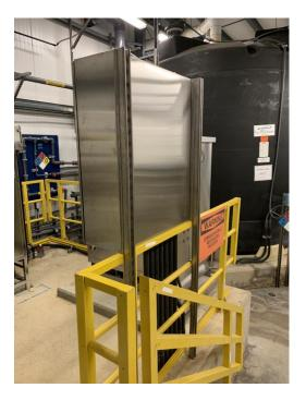
Figure 3.89 – Control Panel not Adequately Braced
