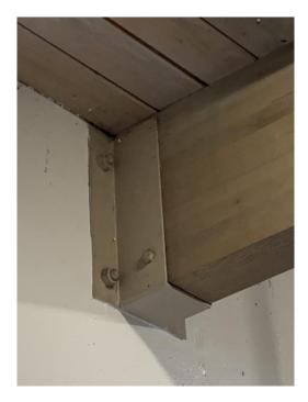
Figure 3.39 – Joist to Perpendicular Wall Connection
