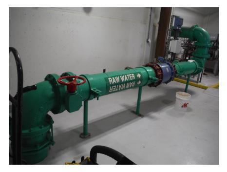
Figure 3.18 – Raw Water Piping System without Adequate Bracing
