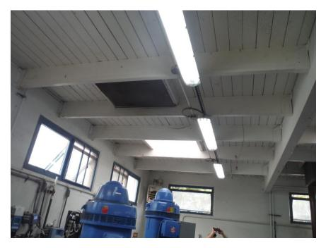
Figure 3.59 – Flexible Diaphragm without Cross Ties
