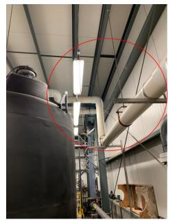
(b) Unbraced Piping Inside the Building
