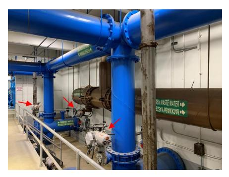
Figure 3.64 – Valves and Valve Actuators Installed In-Line with Piping Systems not Independently Braced
