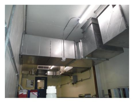
Figure 3.24 – Mechanical Ducts not Braced to Structure
