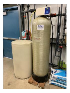
Figure 3.87 – Water Softener Components not Restrained
