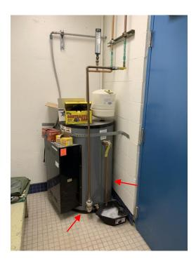
Figure 3.45 – Water Heater Tank not Adequately Restrained
