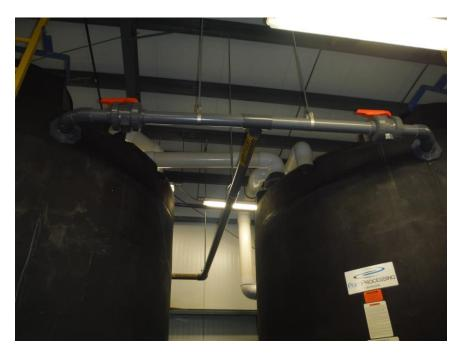
Figure 3.83 – Lack of Flexibility of Piping Connecting Sodium Hypochlorite Tanks
