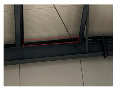
Figure 3.75 – Inadequate Load Path from Roof Diaphragm to Moment Frame Beams (no Blocking between Purlins)
