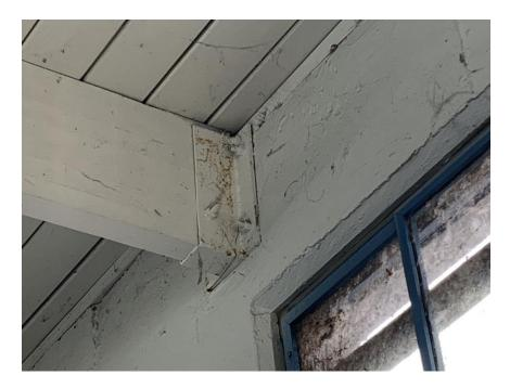
Figure 3.60 – Joist to Perpendicular Wall Connection
