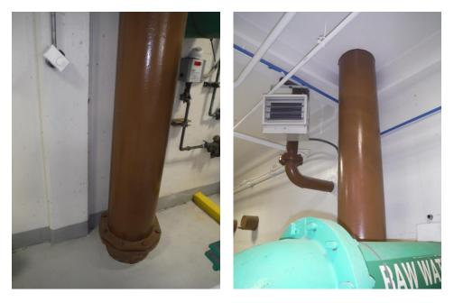
Figure 3.19 – Vertical Pipe without Lateral Restraint
