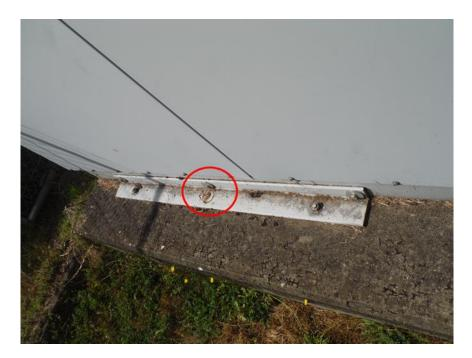
Figure 3.95 – Missing Anchors on Switchgear to Concrete Pad Connection
