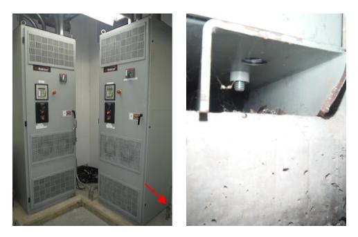
Figure 3.27 – Electrical Cabinets with Missing Anchor at the Base
