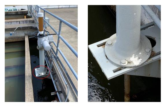
Figure 3.70 – Valve Actuators Installed on Significantly Modified Base Plates
