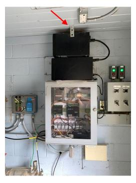
Figure 3.9 – Backup Batteries not Adequately Restrained
