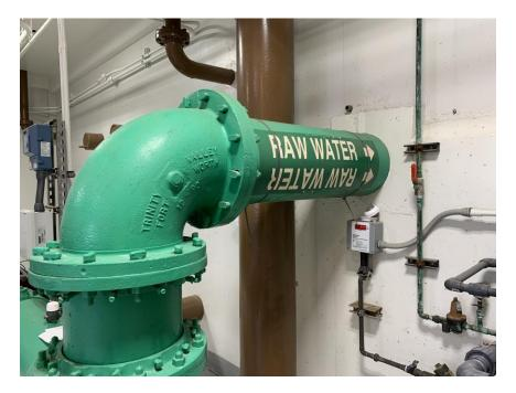
Figure 3.17 – Concrete Wall Penetration by Raw Water Pipe
