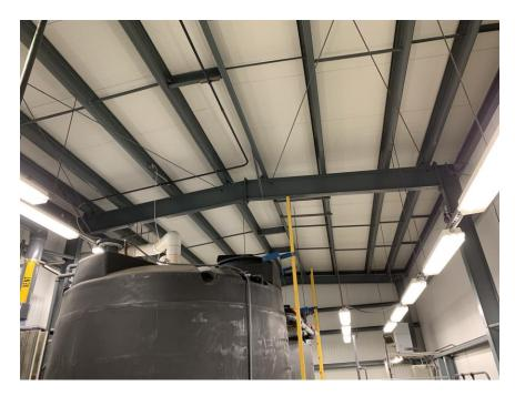
Figure 3.74 – Single Lateral Force Resisting Bay in Frame Line along North-South Direction
