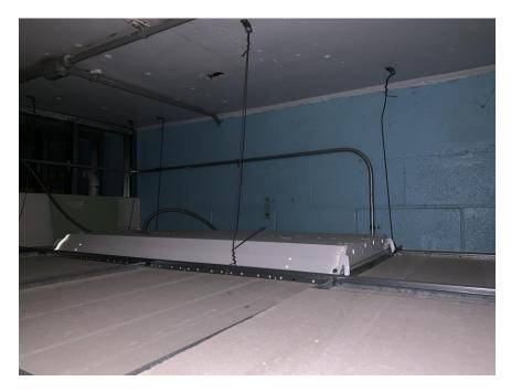
Figure 3.46 – Light Fixture Supported by Ceiling Grid
