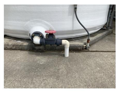
Figure 3.81 – Lack of Flexibility in Salt Brine Tank Drain Pipe
