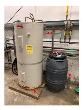
Figure 3.86 – Water Heater not Adequately Restrained and Unrestrained Barrel
