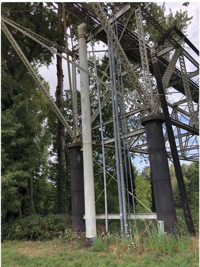
Figure 2. 24-inch Water Transmission Main
