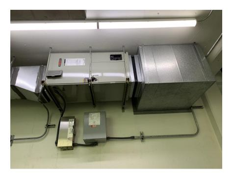
Figure 3.25 – In-Line Fan Unit Unrestrained to Movement Parallel to Wall
