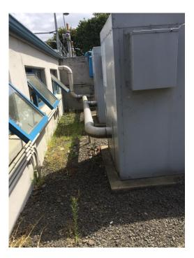
Figure 3.65 – Air Scour Piping from Blowers to Filter Gallery without Adequate Flexibility to Accommodate Differential Movement
