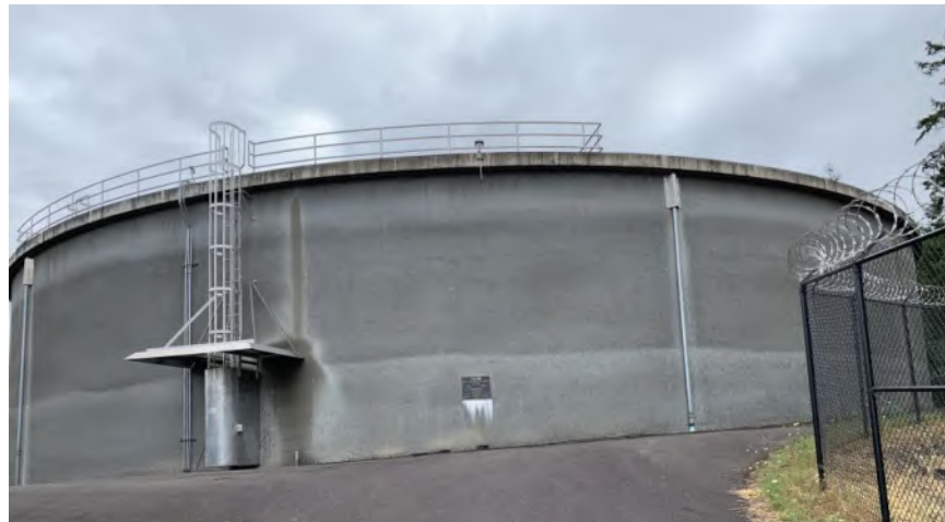
Figure 3.1 – Corral Creek Road Reservoir
