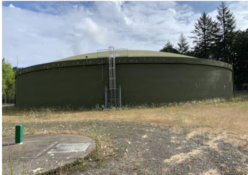
Figure 3.11 – North Valley Reservoir No.2
