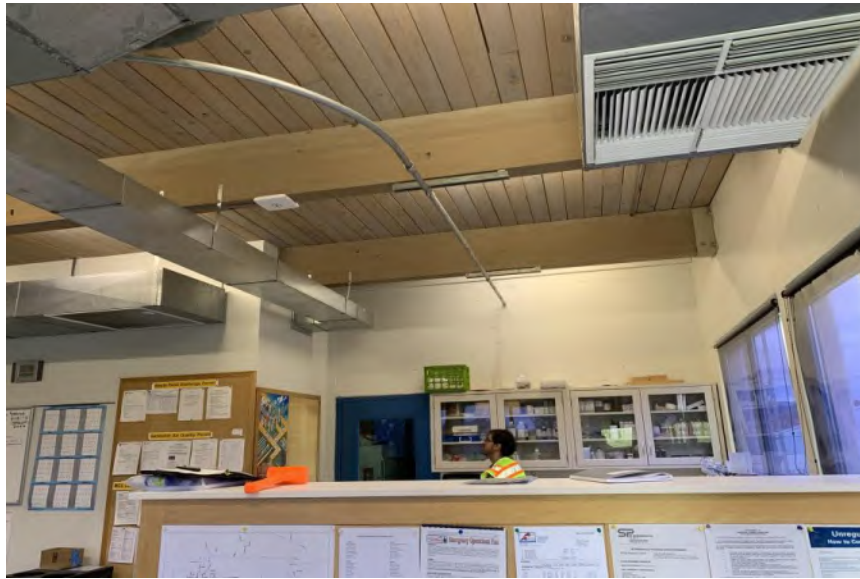
Figure 3.38 – Flexible Diaphragm Chords without Cross Ties
