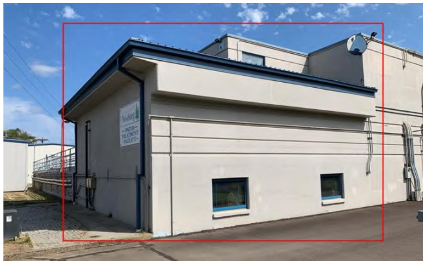
Figure 3.31 – 1961 Treatment/Control Building Addition
