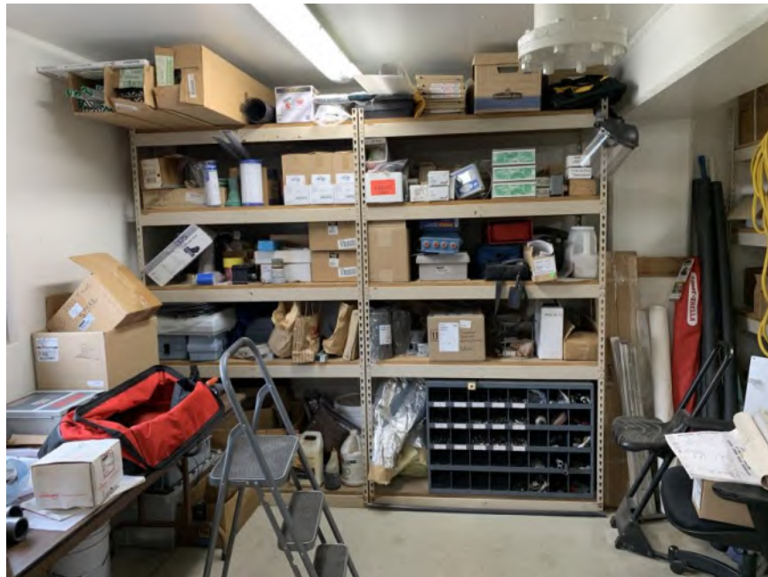
Figure 3.33 – Unrestrained Storage Rack
