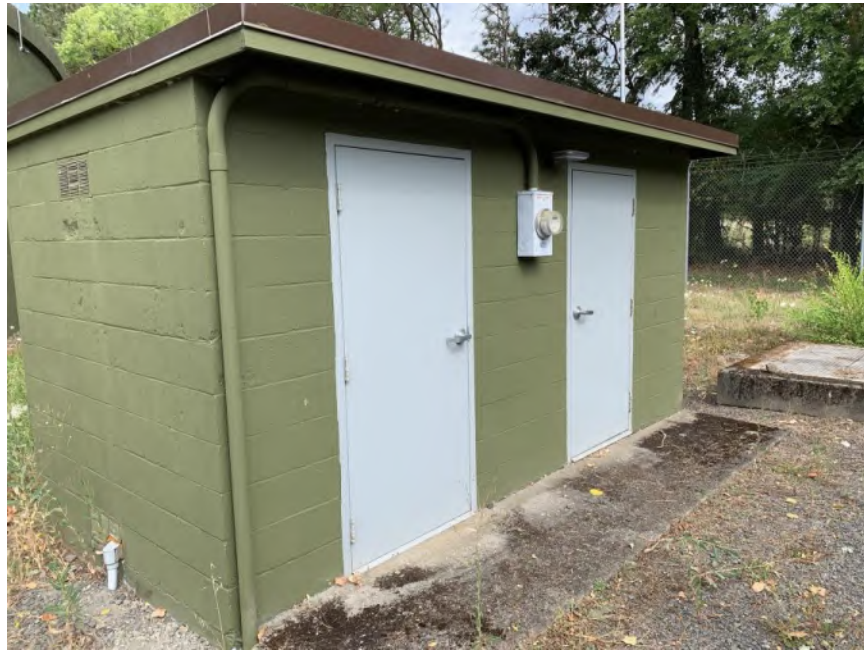
Figure 3.6 – Former Chlorination Building
