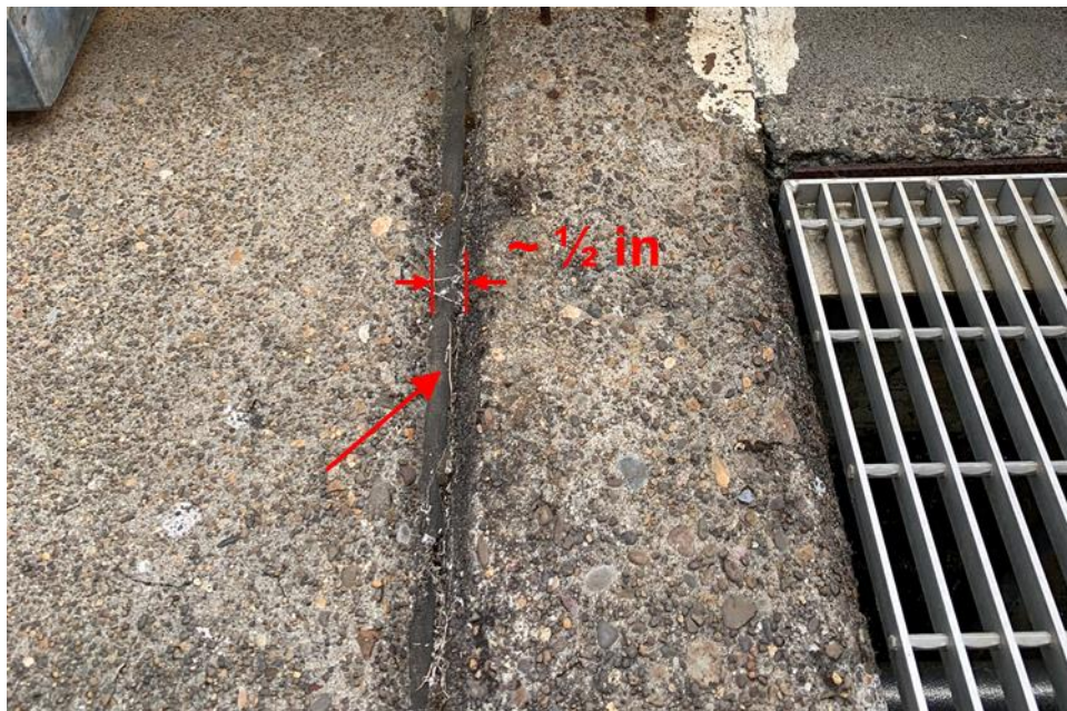
Figure 3.48 – Construction Joint Between Sedimentation Basins No. 1 (1961 Construction) and No. 2 (pre-1961 Construction)
