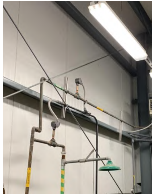
(b) West Bay with Rod Bracing
