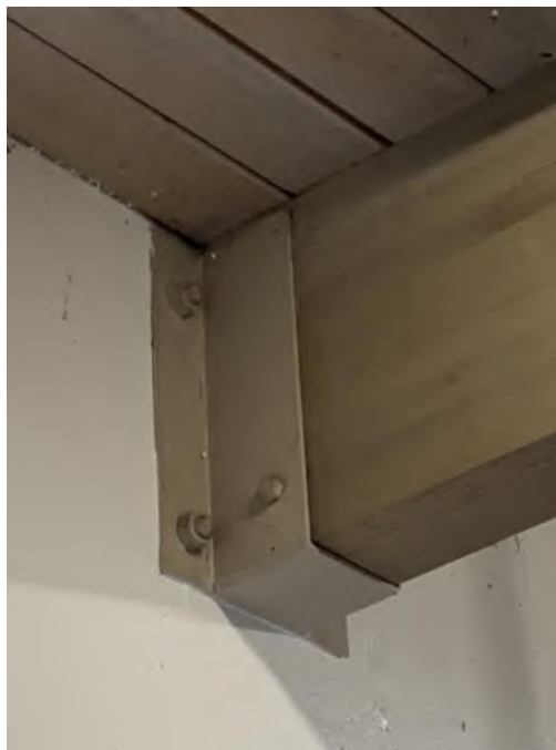
Figure 3.39 – Joist to Perpendicular Wall Connection
