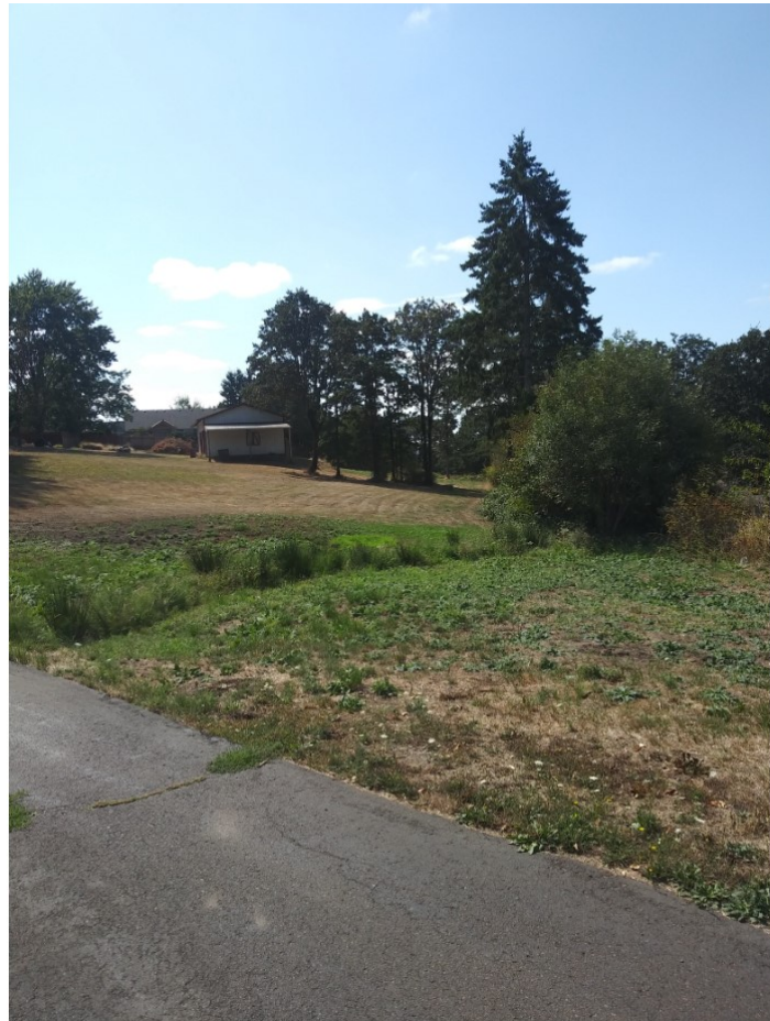
Figure 4: Swale Discharge Channel
