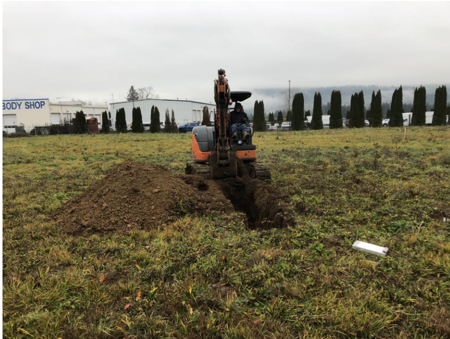
Test Pit TP-4
