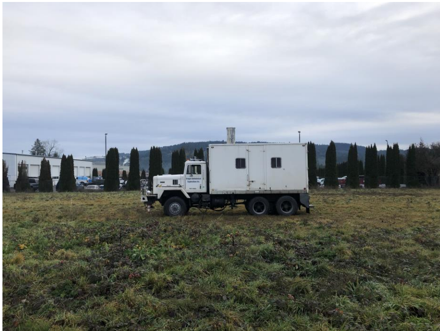
Cone Penetrometer Testing
