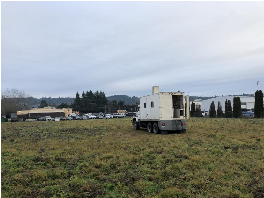
Cone Penetrometer Testing
