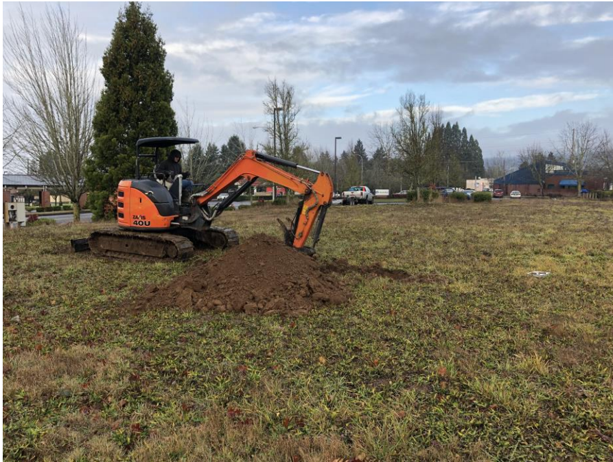
Test Pit TP-1
