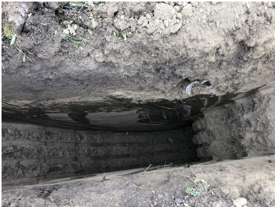
Test Pit TP-4
