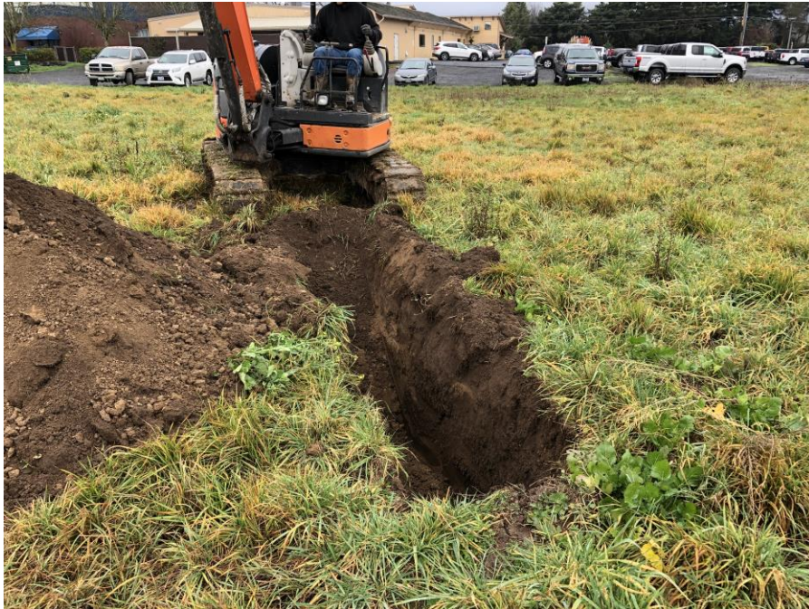
Test Pit TP-3
