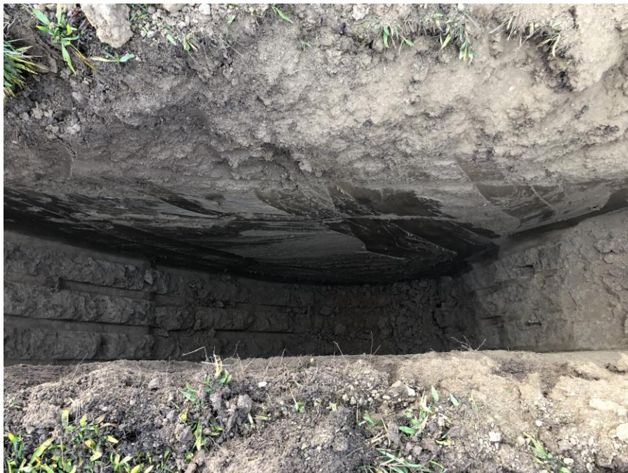
Test Pit TP-1
