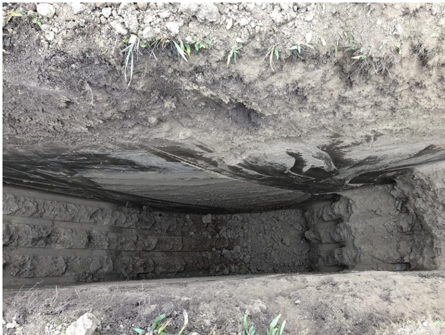
Test Pit TP-2
