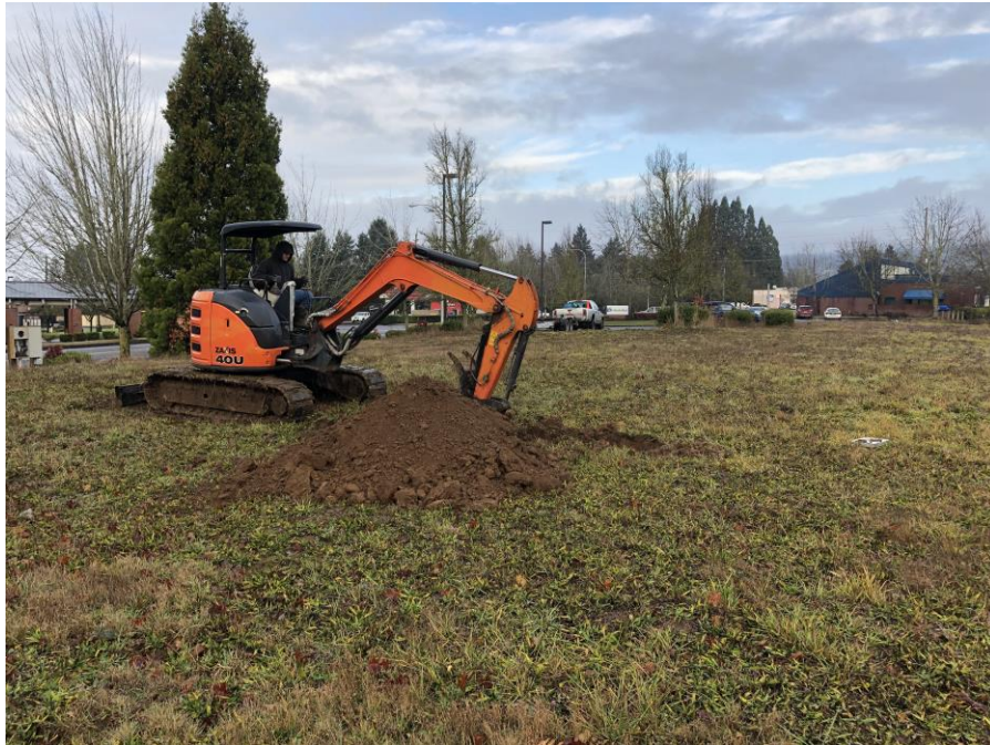
Test Pit TP-1
