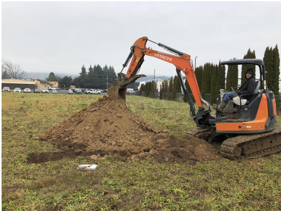
Test Pit TP-2
