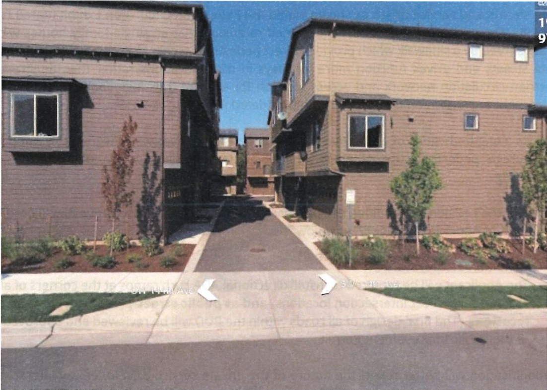
Photo 2: Private Service Drive/Driveway at Public Street
