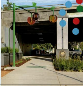
Many sidewalks and roadways need improvement in the project area. Especially under the bypass, creating active, welcoming space will improve mobility between the riverfront and downtown.
