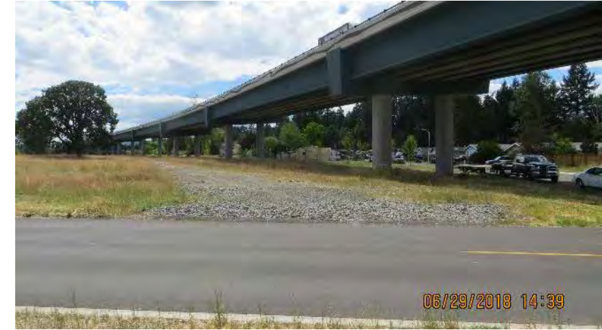
College Street passing under Bypass
