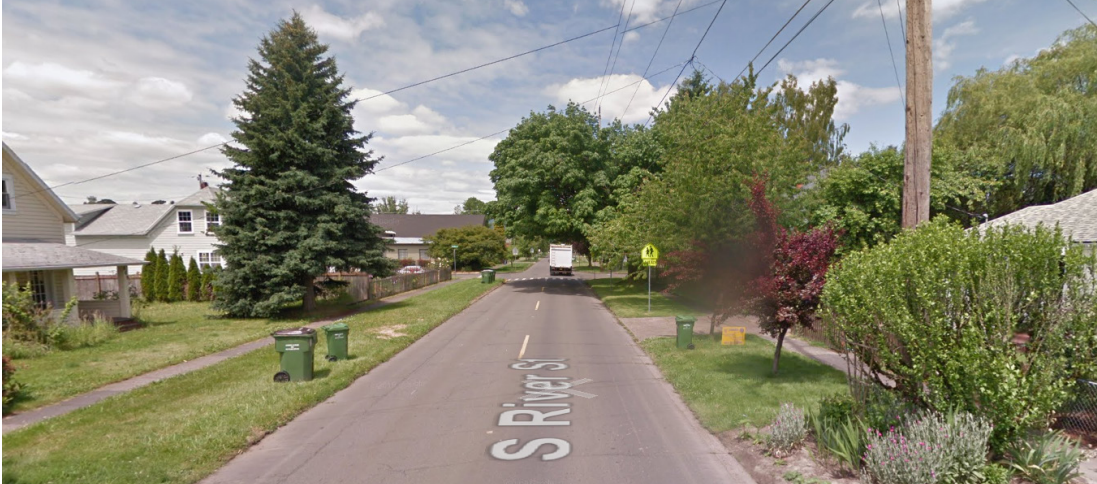
S RIVER STREET NORTH OF E NINTH STREET (LOOKING NORTH) - 60' ROW
