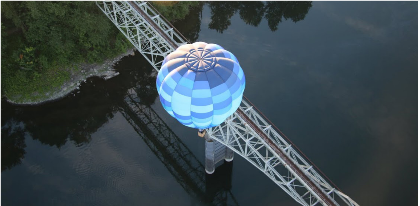
FIGURE 24. VIEW OF WATERLINE BRIDGE, A POTENTIAL LOCATION FOR A BICYCLE/PEDESTRIAN CROSSING OF THE WILLAMETTE
