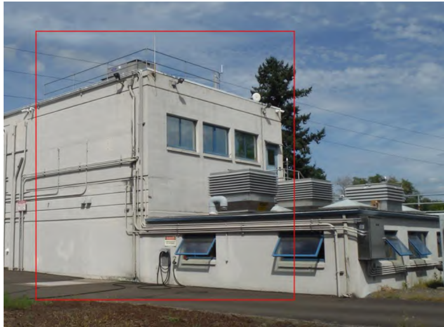
Figure 3.36 – 1970 Treatment/Control Building Addition
