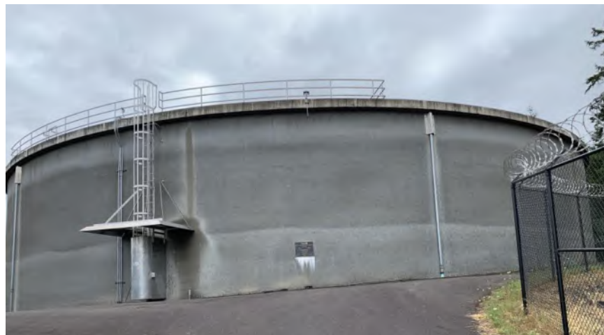
Figure 3.1 – Corral Creek Road Reservoir
