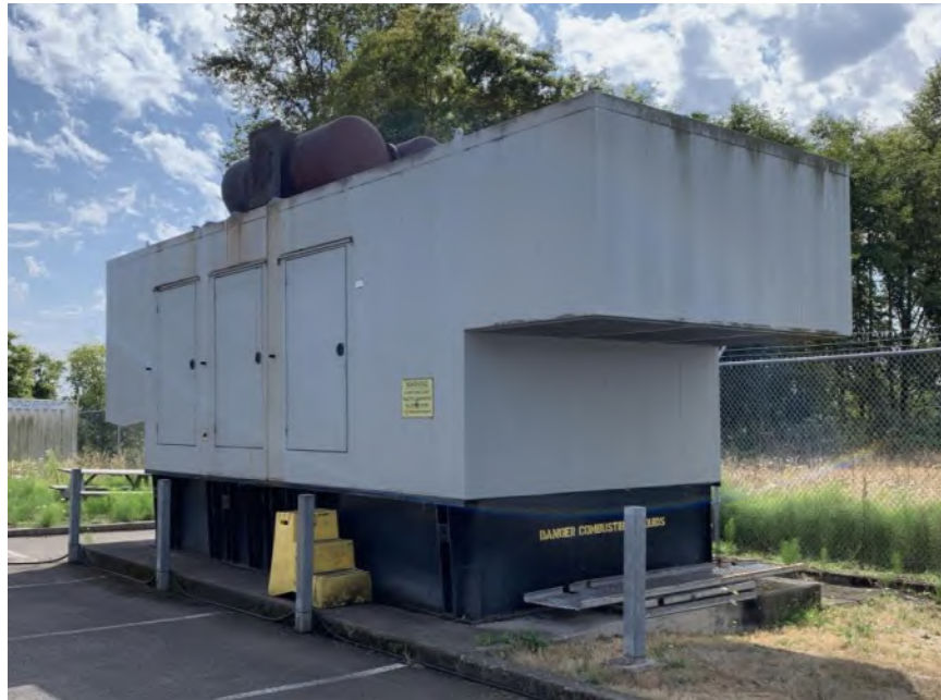
Figure 3.92 – Emergency Generator
