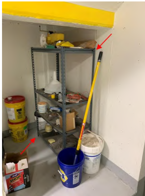
Figure 3.23 – Unrestrained Storage Rack
