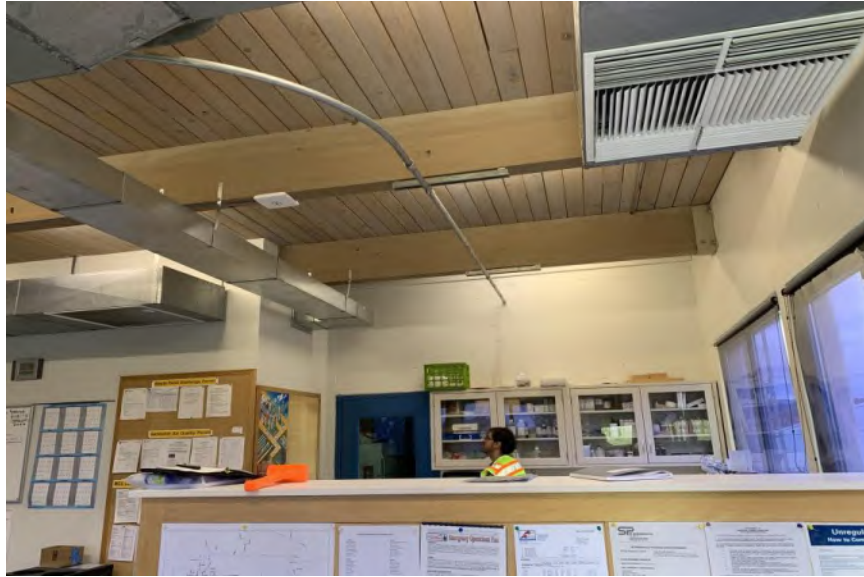
Figure 3.38 – Flexible Diaphragm Chords without Cross Ties
