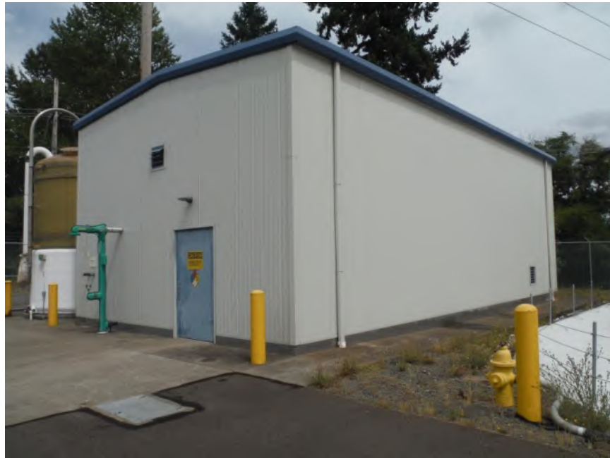
Figure 3.71 – Sodium Hypochlorite Generation Building
