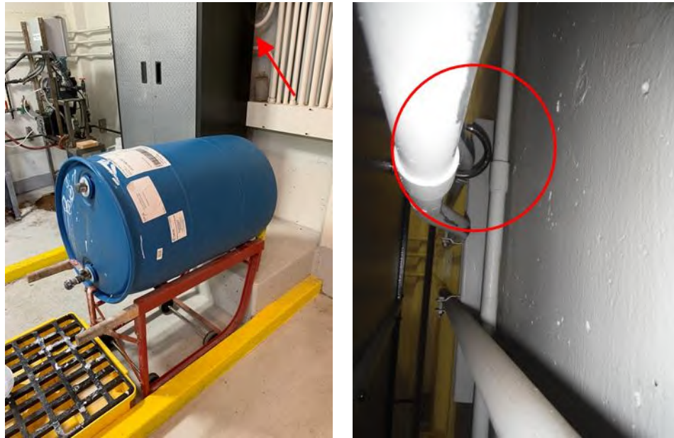
Figure 3.22 – Storage Cabinet Restrained with U-Bolt to Electrical Conduits
