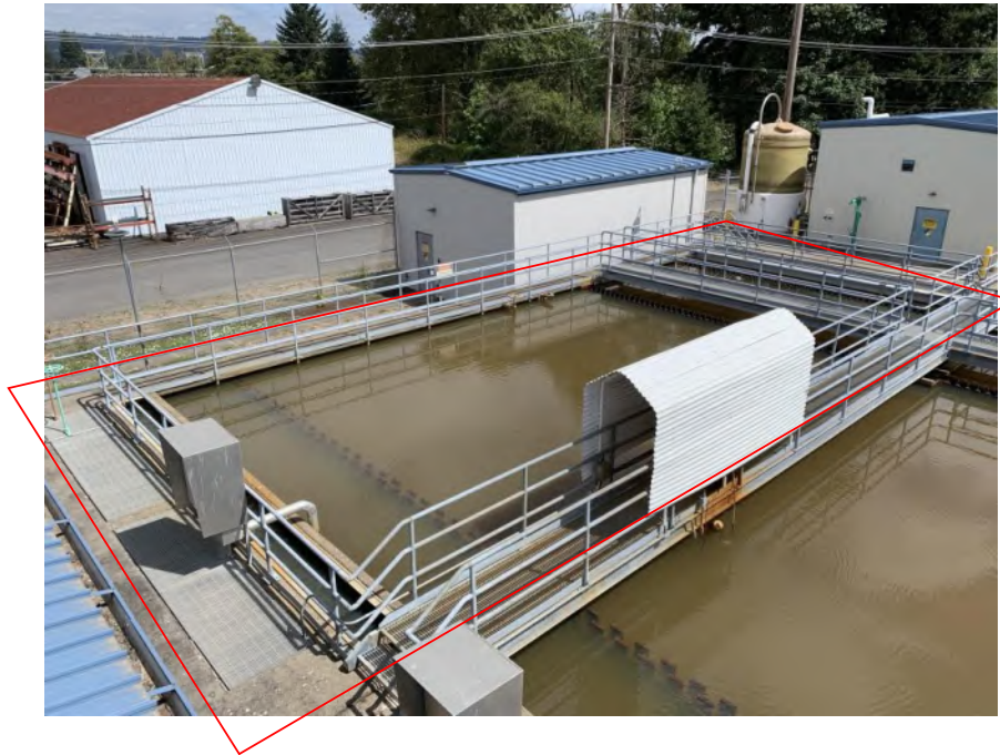
Figure 3.47 – Sedimentation Basin No. 1 Structure
