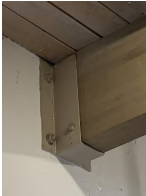
Figure 3.39 – Joist to Perpendicular Wall Connection
