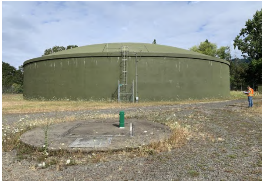
Figure 3.4– North Valley Reservoir No. 1
