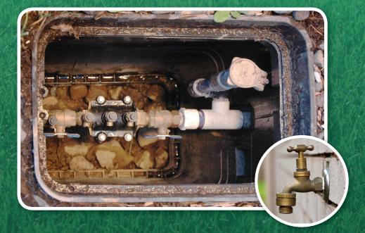
What's a Backflow Device? Do I have a Device? The sprinkler system or water fountain at your home should have a backflow prevention device on it. This device prevents water that has entered the fountain or sprinklers from accidentally flowing back into the drinking water lines.
