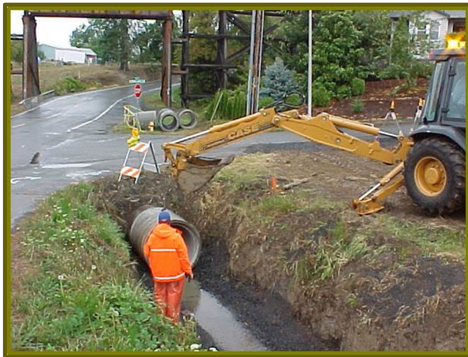
Villa Road Drainage Pipe Installation
