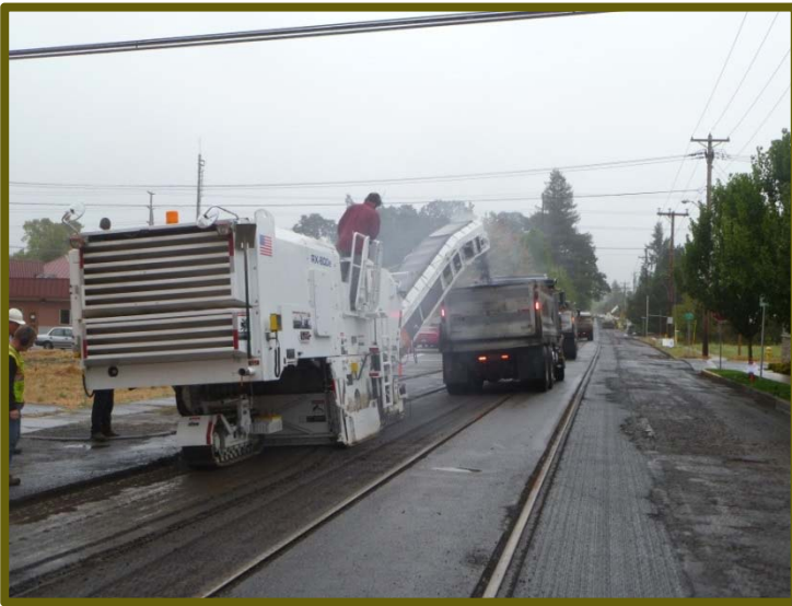
2012: Removal of existing Pavement on Blaine St.
