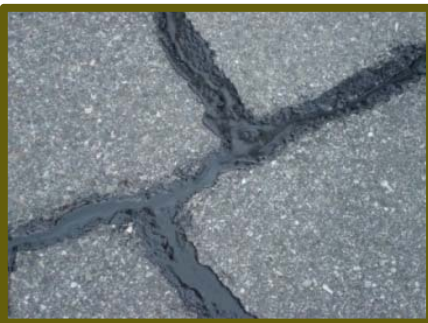
Crack Seal
