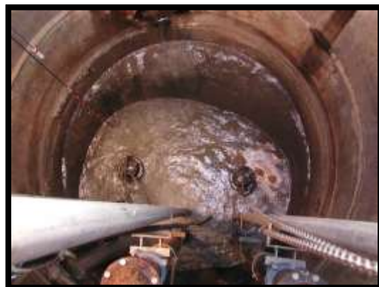
FIGURE 16 INFLOW & INFILTRATION AT THE FERNWOOD & CREEKSIE LIFT STATION
