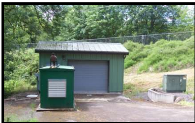
FIGURE 19 DAYTON AVE LIFT STATION (LEFT) & GORMAN- RUPP TOP-SIDE DRY LIFT (RIGHT)
