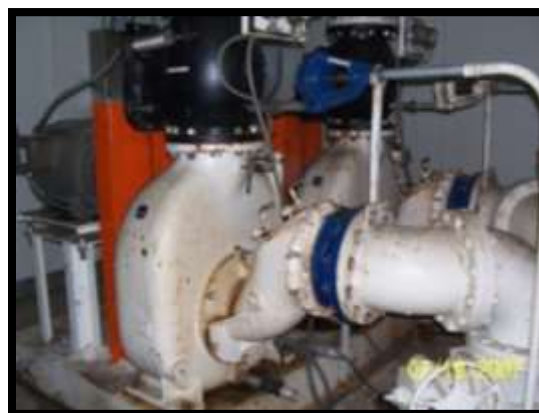
FIGURE 19 DAYTON AVE LIFT STATION (LEFT) & GORMAN- RUPP TOP-SIDE DRY LIFT (RIGHT)
