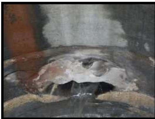
FIGURE 16 INFLOW & INFILTRATION AT THE FERNWOOD & CREEKSIE LIFT STATION
