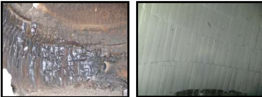
FIGURE 14 DEHYDRATION UNIT BURNER BEFORE AND AFTER CONDITION
