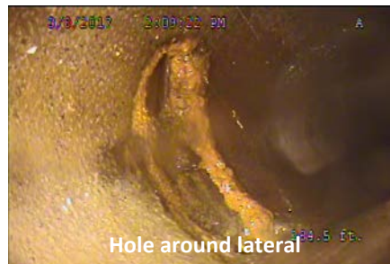
Large hole around lateral
