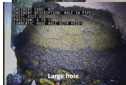
Separated joint with void visible
