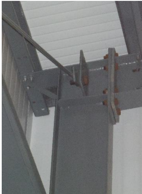
Figure 3.77 – View of Moment Frame Connection and Panel Zone
