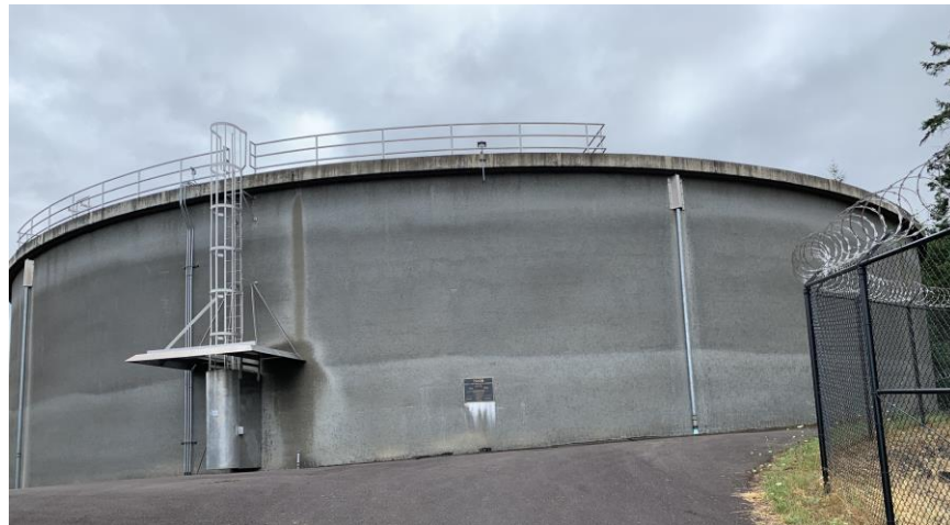
Figure 3.1 – Corral Creek Road Reservoir
