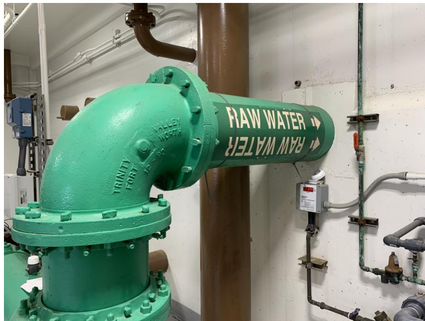
Figure 3.17 – Concrete Wall Penetration by Raw Water Pipe
