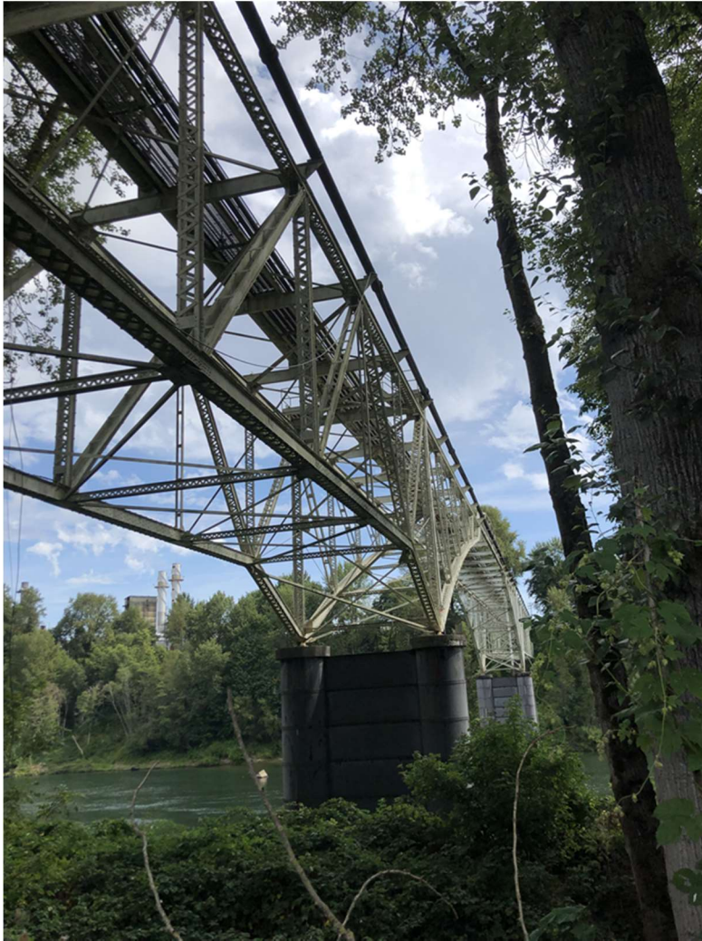
Figure 1. Pipeline Bridge Superstructure
