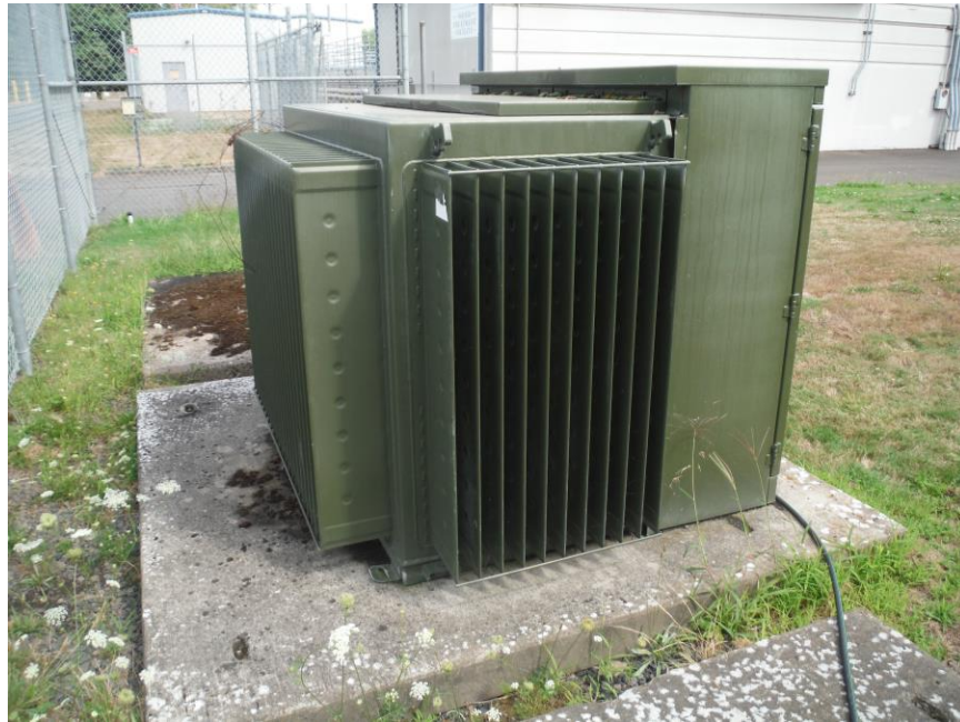
Figure 3.94 – Electrical Transformer
