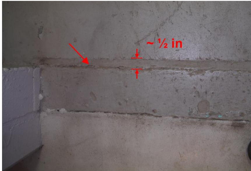
Figure 3.16 – Seismic Joint Between Original Treatment/Control Building (pre-1961) and 1961 Addition
