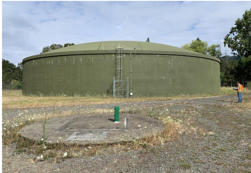
Figure 3.4 – North Valley Reservoir No. 1
