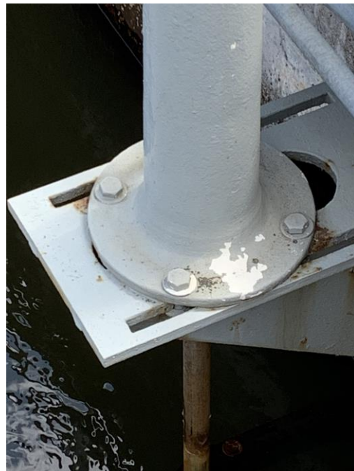
Figure 3.70 – Valve Actuators Installed on Significantly Modified Base Plates
