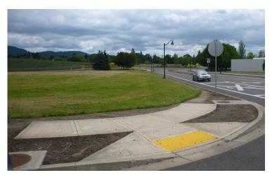
ADA Compliant Curb Ramp with No Connections
