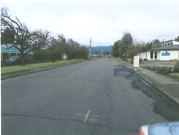
Photo 1: Deborah Road leading from 99W towards Newberg Schools and sports complexes. Classified as a Minor Collector. Needs dedicated bike lanes. Has no need of on-street parking. Note that it does not have planter strips.
