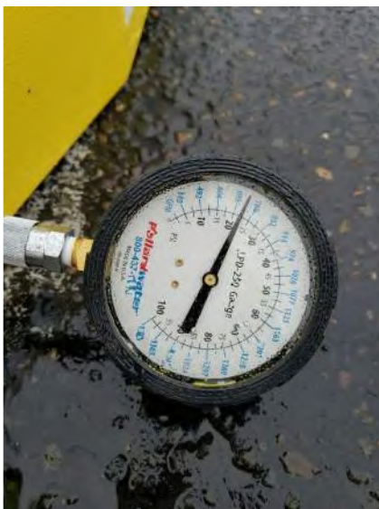
Pitot reading with dechlor diffuser on flowed hydrant located on Fulton Street and East Cherry Street
