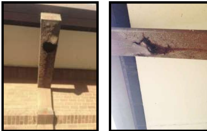
FIGURE 18 ROOF MAINTENANCE AT WASTEWATER TREATMENT PLANT
