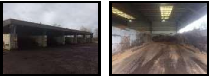
FIGURE 14 EXISTING CURING BAYS
