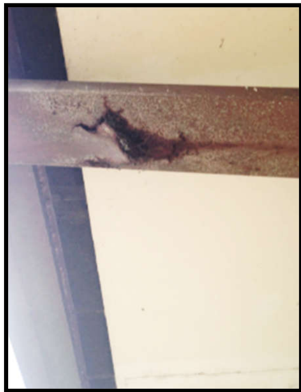
FIGURE 10 ROOF MAINTENANCE AT WASTEWATER TREATMENT PLANT
