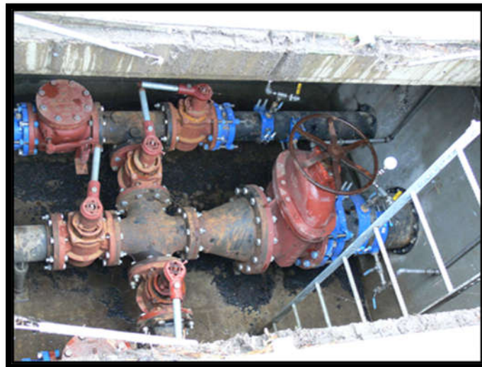
FIGURE 16 FERNWOOD VALVE VAULT
