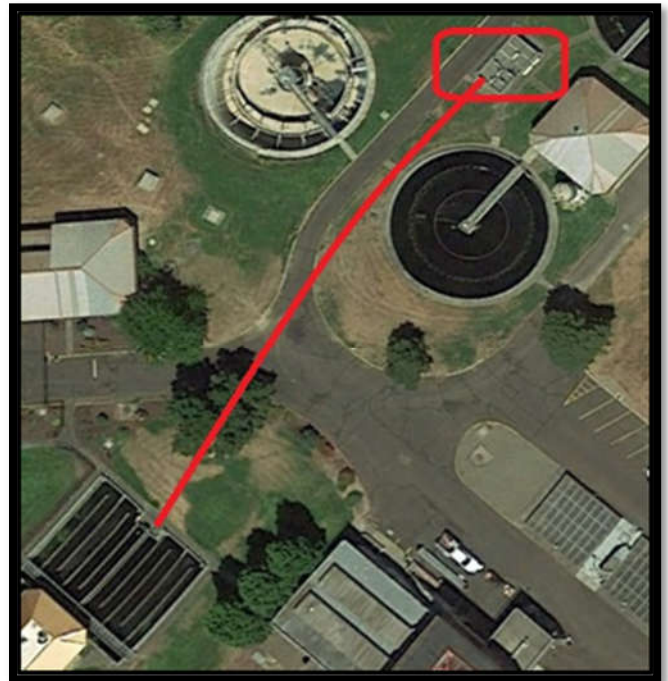
FIGURE 18 INSTALLATION OF A SECOND (PARALLEL) PIPE FROM THE CLARIFIER EFFLUENT TO THE CHLORINE CONTACT BASIN
