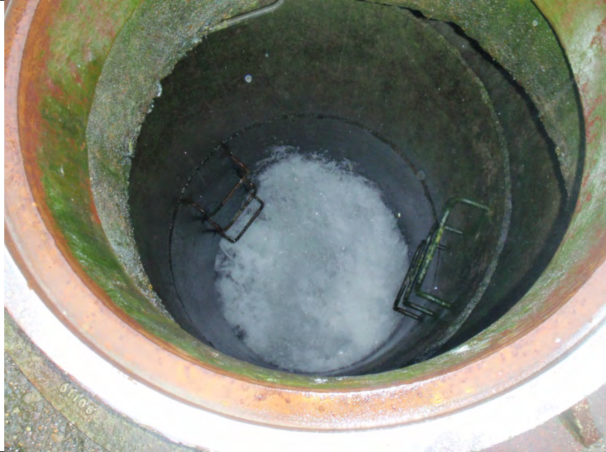
Photo 2 – Inside manhole at approximately 8 mgd
