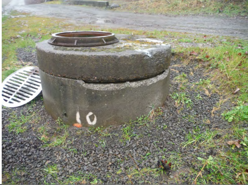
Photo 1 – Outfall final manhole
