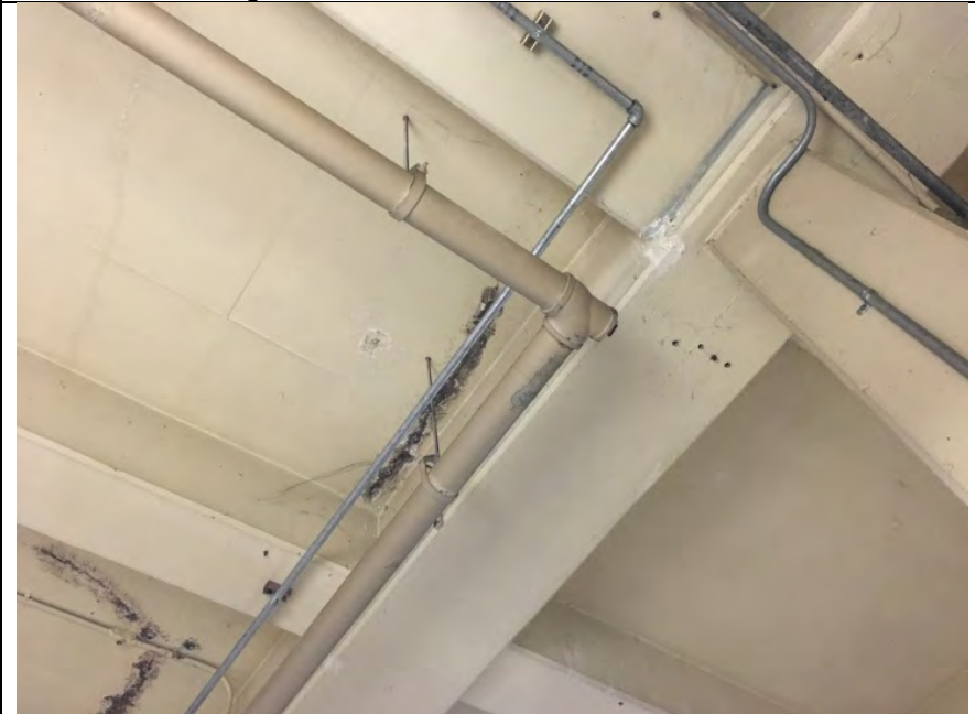
Photo 2 – Ceiling Cracks
