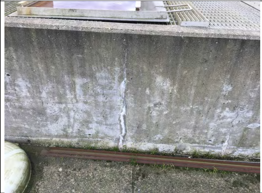
Photo 2 – Wall Crack
