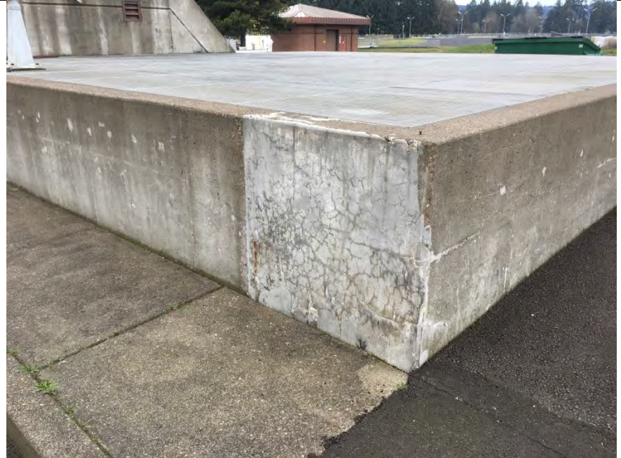
Photo 4 – Concrete Spalling
