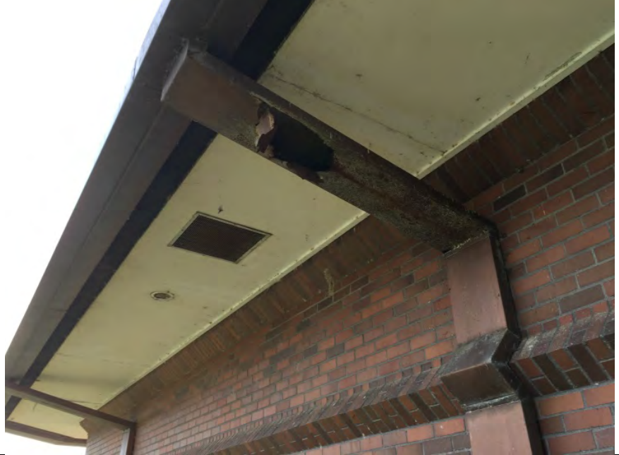
Photo 2 – Gutter Corrosion
