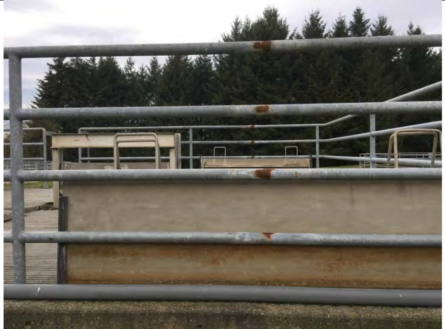
Photo 2 – Handrail Corrosion
