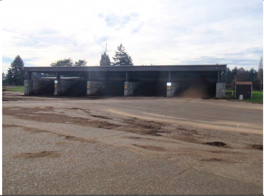
Photo 1 – Compost Curing Bays
