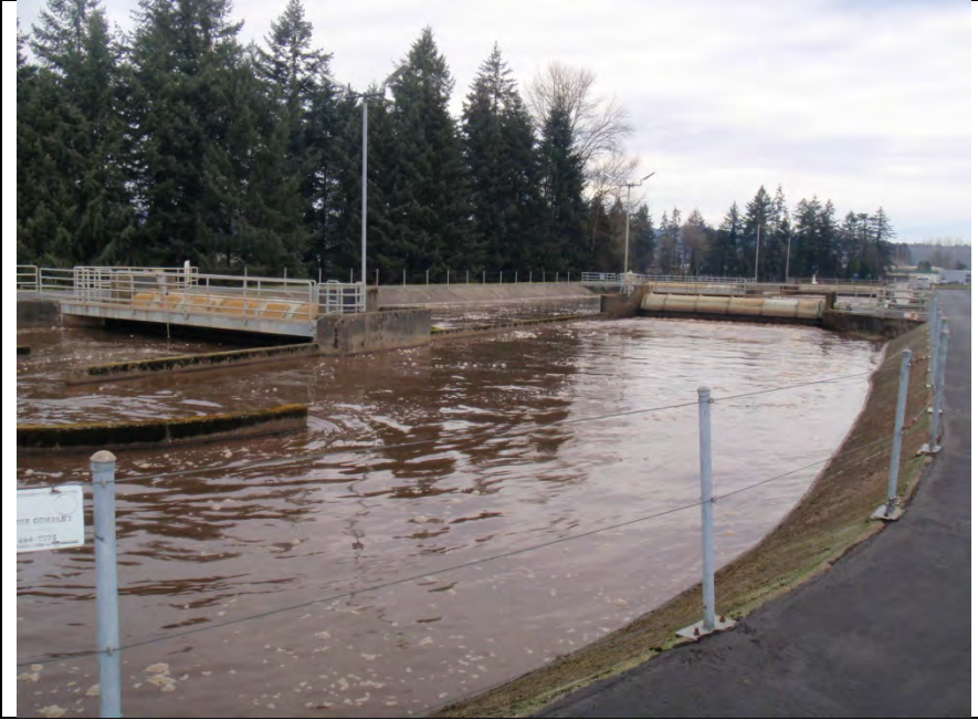
Photo 1 – Oxidation Ditch 1
