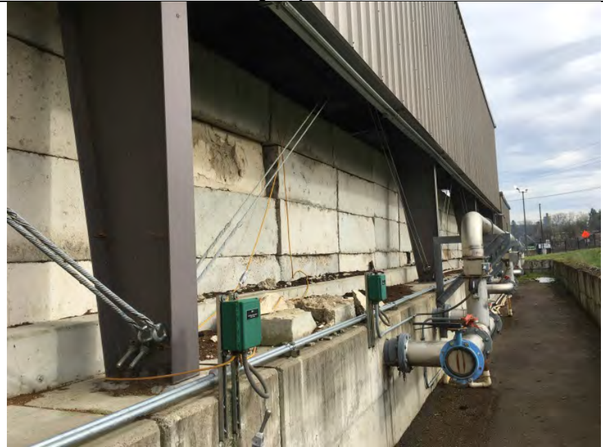
Photo 4 – Backside of Curing Bays
