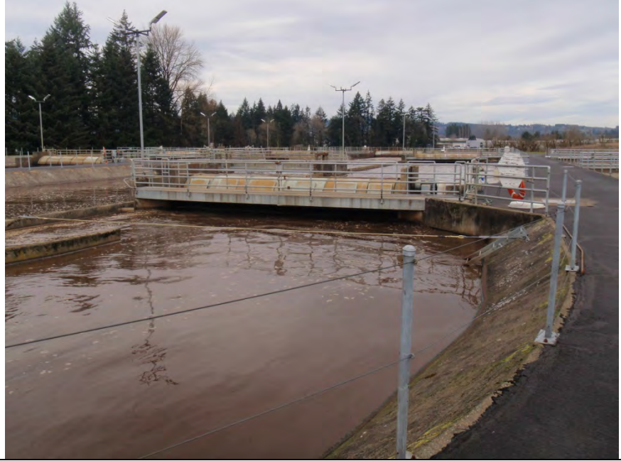
Photo 1 – Oxidation Ditch 2
