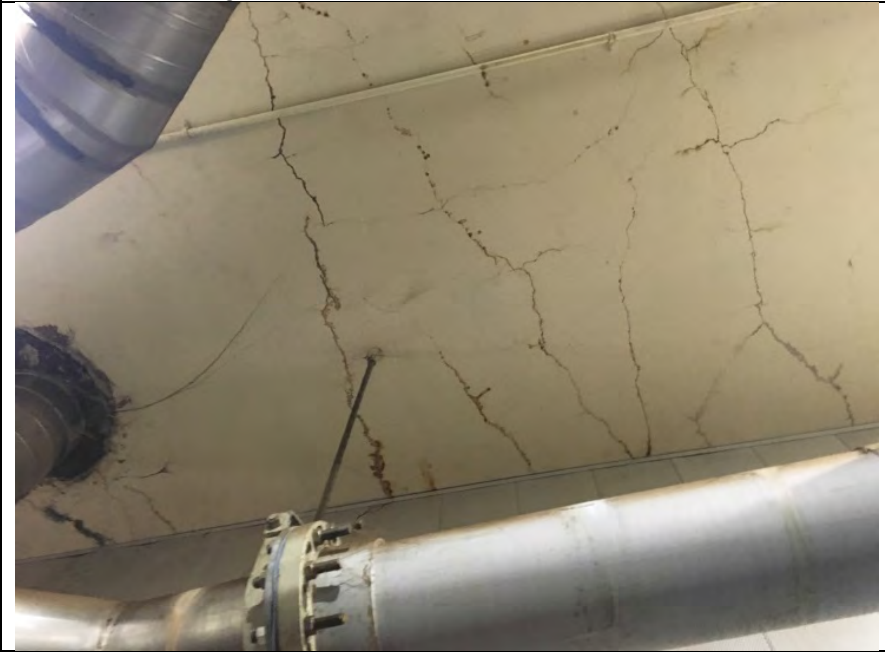
Photo 8 – Ceiling Cracks 1
