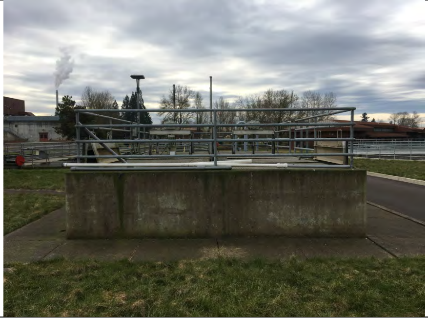
Photo 1 – Clarifier Distribution Box
