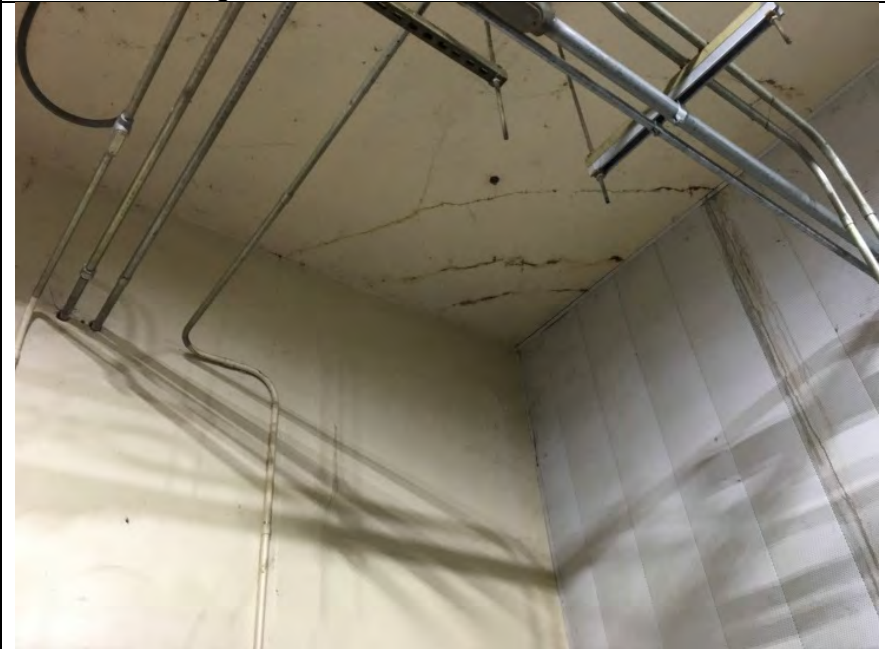
Photo 9 - Ceiling Cracks 2
