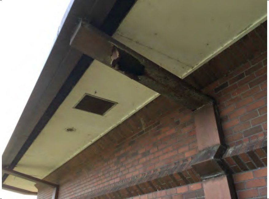
Photo 2 – Gutter Corrosion
