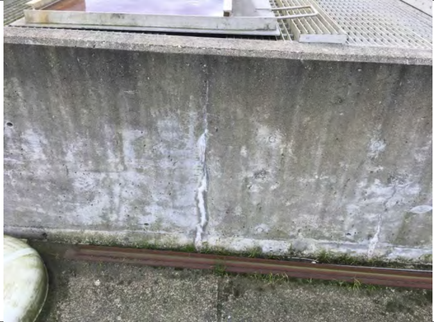
Photo 2 – Wall Crack
