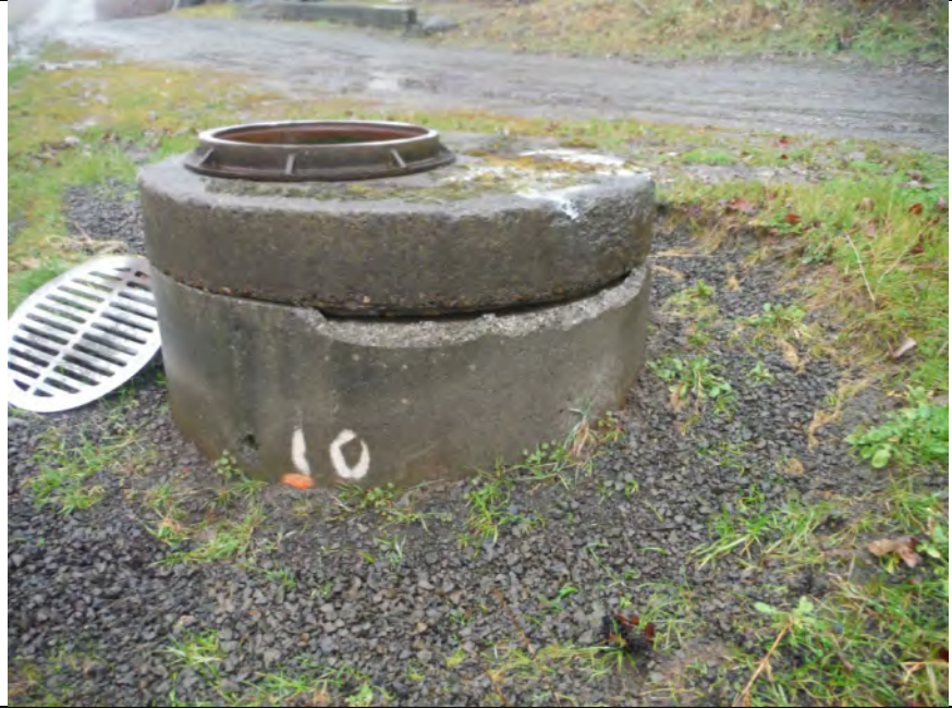
Photo 1 – Outfall final manhole
