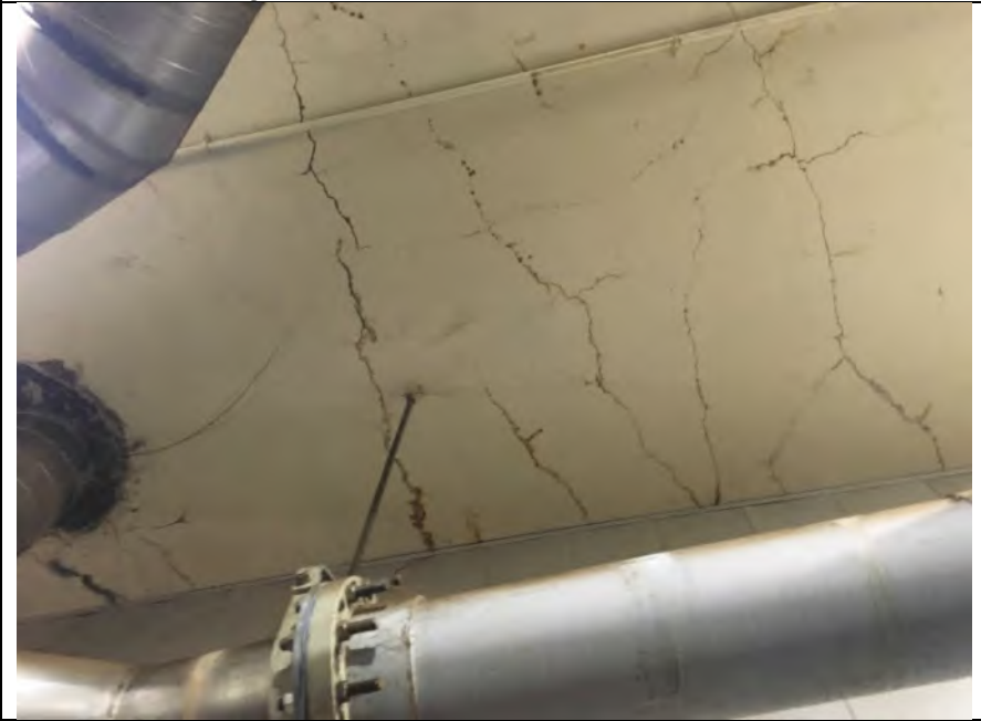
Photo 8 – Ceiling Cracks 1
