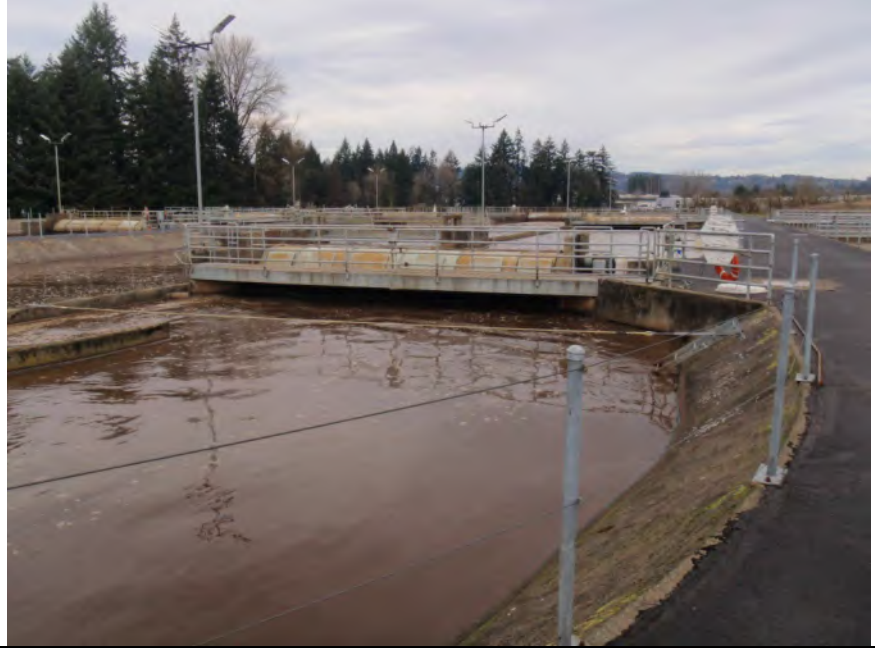
Photo 1 – Oxidation Ditch 2
