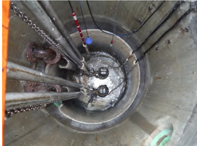
Creekside Lift Station
