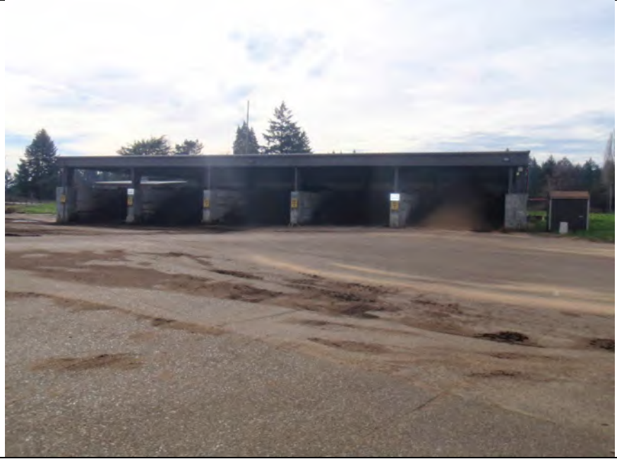
Photo 1 – Compost Curing Bays
