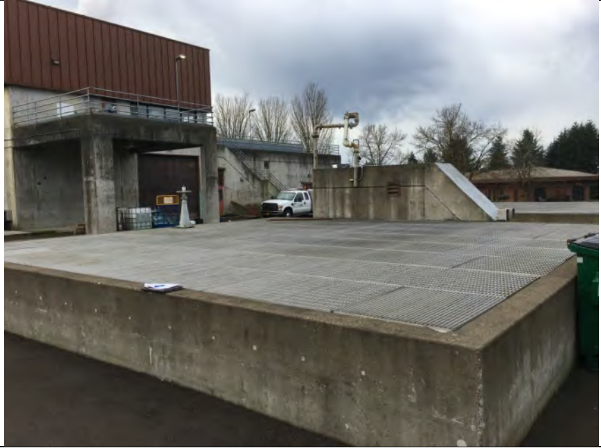
Photo 1 – Sludge Storage Tanks
