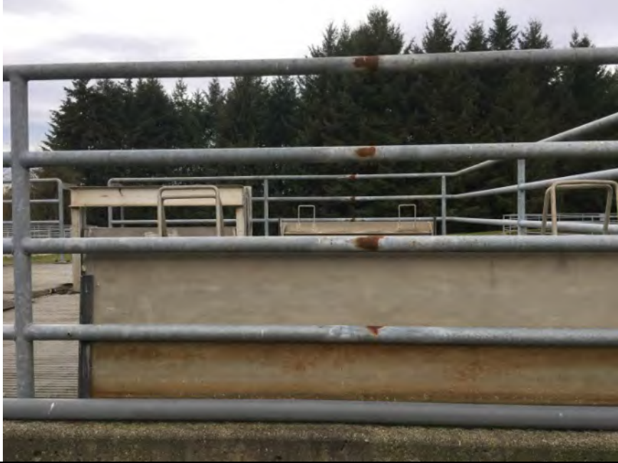
Photo 2 – Handrail Corrosion
