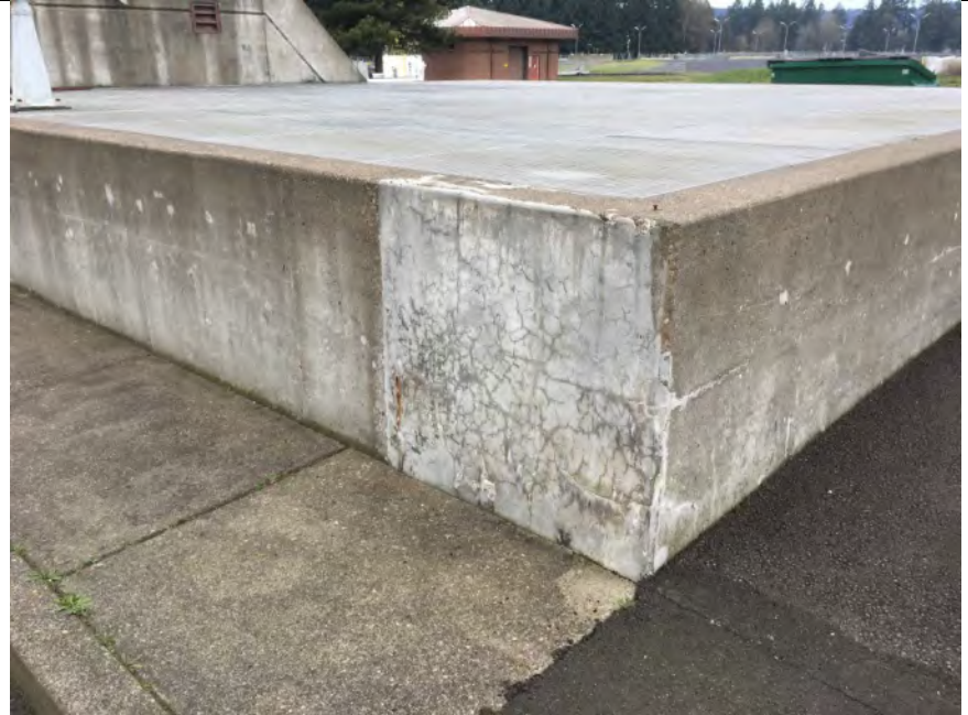
Photo 4 - Concrete Spalling
