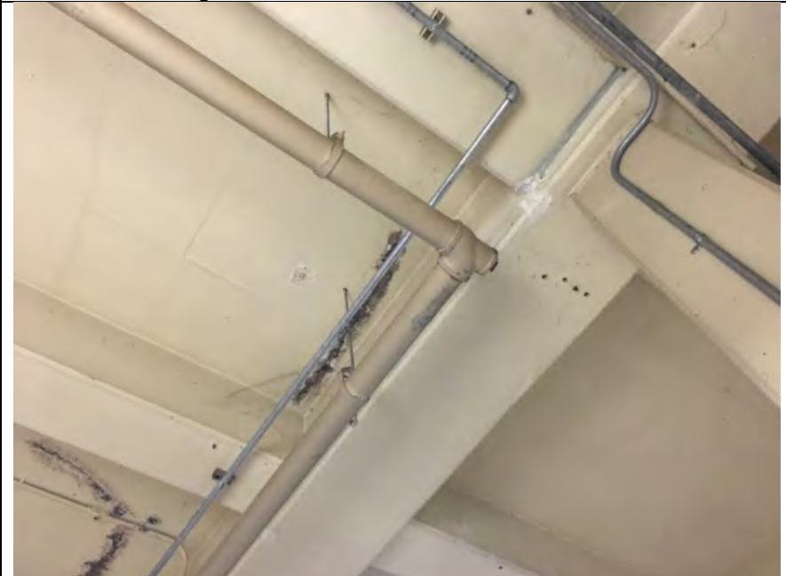
Photo 2 – Ceiling Cracks
