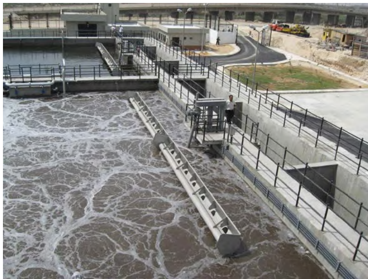
Figure 10-7: Example of SBR Installation
