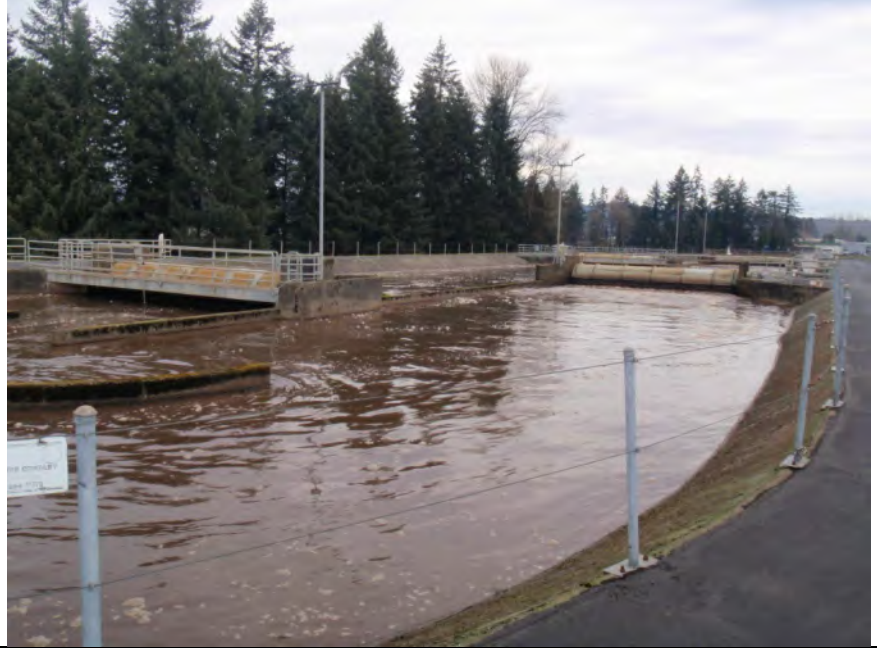
Photo 1 – Oxidation Ditch 1
