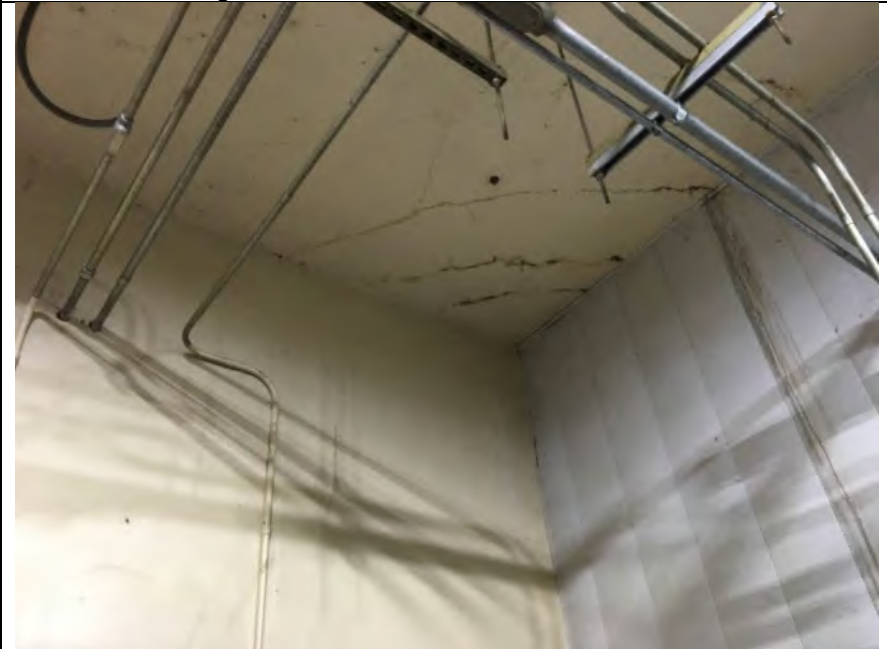
Photo 9 - Ceiling Cracks 2
