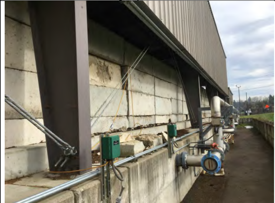
Photo 4 – Backside of Curing Bays
