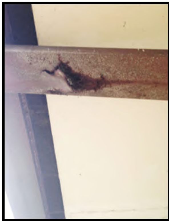
FIGURE 10 ROOF MAINTENANCE AT WASTEWATER TREATMENT PLANT
