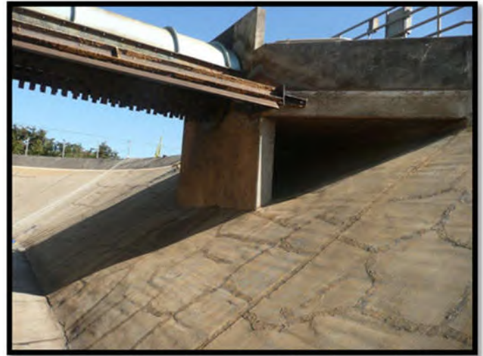
FIGURE 9 OXIDATION DITCH
