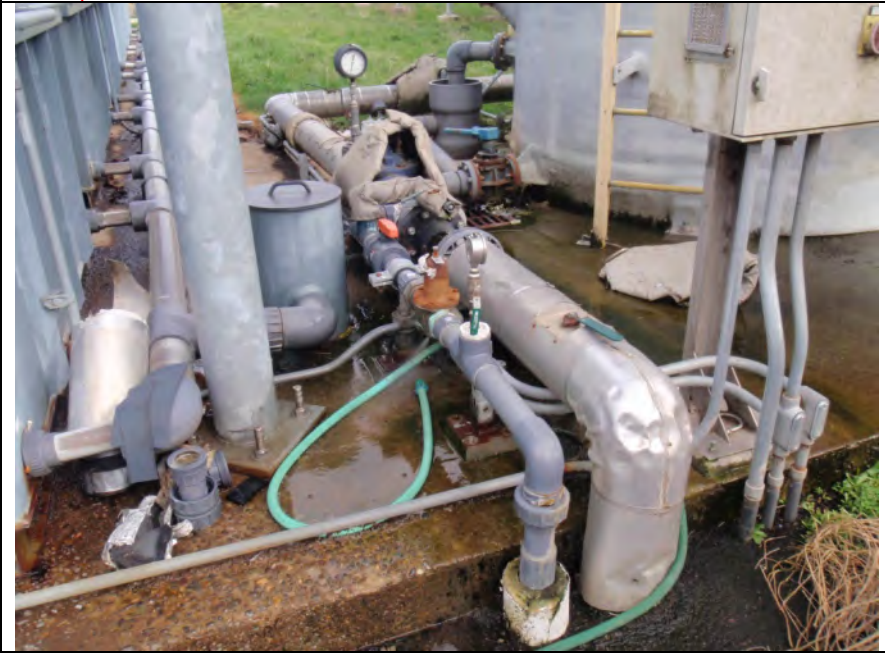
Photo 3 – Piping (Water piping improvements made in Summer 2017)
