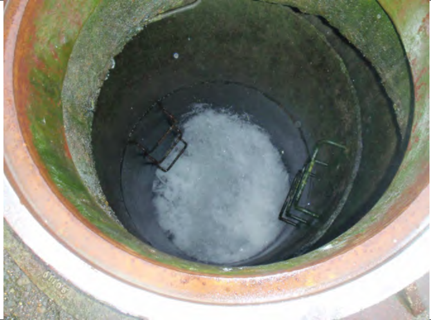
Photo 2 – Inside manhole at approximately 8 mgd
