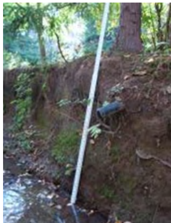
Example photos of stream reach below Mountainview Drive. Residential drainage pipes enter channel on west side.
