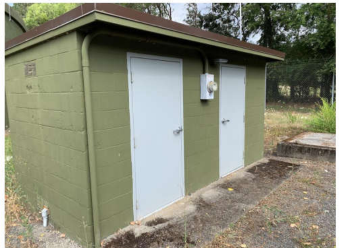
Figure 3.6 – Former Chlorination Building
