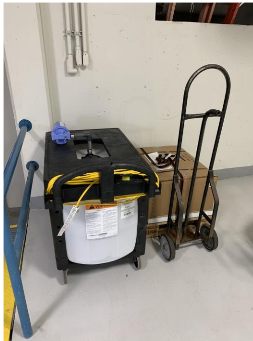
Figure 3.21 – Unrestrained Rolling Carts
