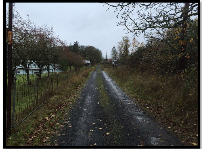
FIGURE 31 NORTH VALLEY RESERVOIR ACCESS ROAD
