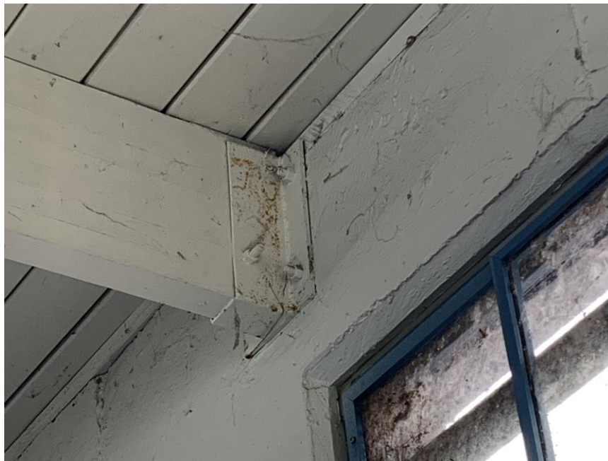
Figure 3.60 – Joist to Perpendicular Wall Connection
