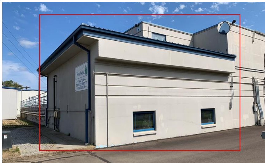
Figure 3.31 – 1961 Treatment/Control Building Addition
