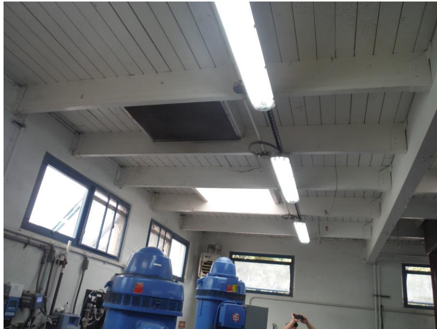
Figure 3.59 – Flexible Diaphragm without Cross Ties
