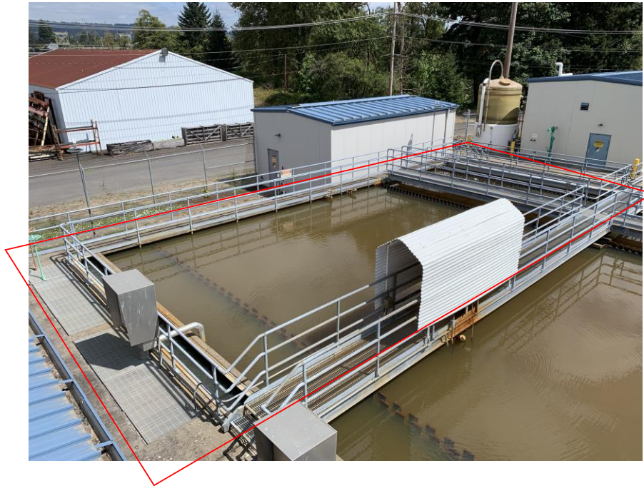
Figure 3.47 – Sedimentation Basin No. 1 Structure
