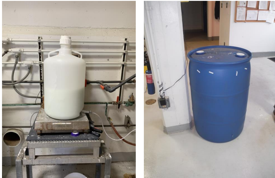
Figure 3.20 – Unrestrained Chemical Storage Containers
