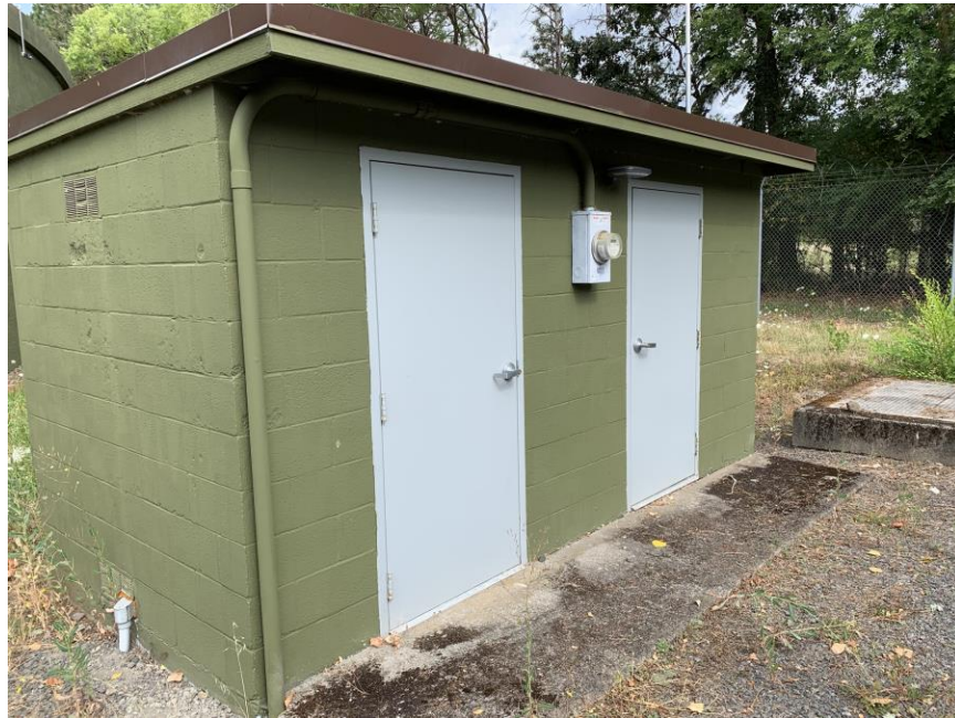
Figure 3.6 – Former Chlorination Building
