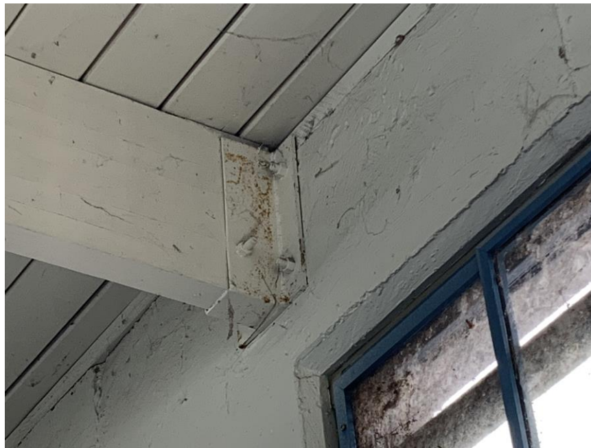
Figure 3.60 – Joist to Perpendicular Wall Connection
