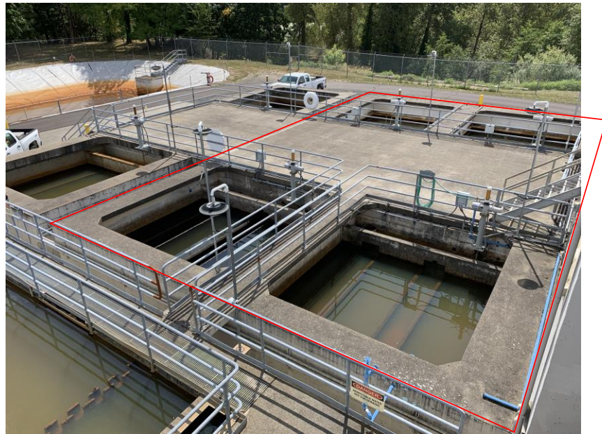
Figure 3.54 – Filters No. 1 to 4 and Filter Gallery Roof Slab
