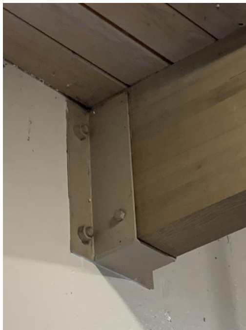
Figure 3.39 – Joist to Perpendicular Wall Connection
