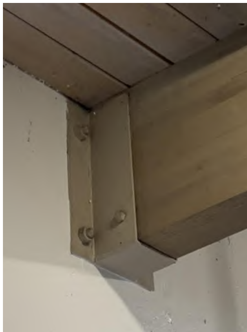
Figure 3.39 – Joist to Perpendicular Wall Connection
