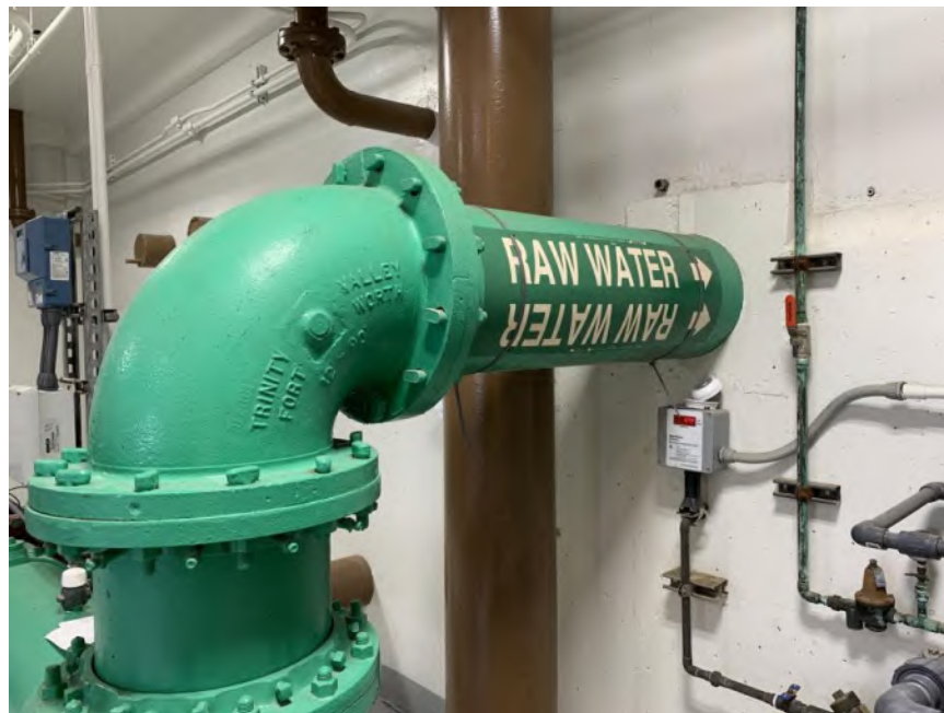
Figure 3.17 – Concrete Wall Penetration by Raw Water Pipe
