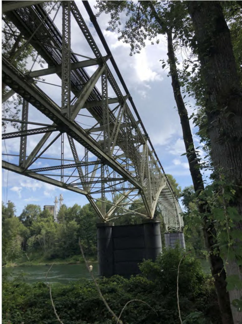
Figure 1. Pipeline Bridge Superstructure
