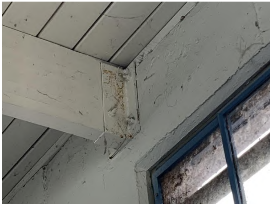
Figure 3.60 – Joist to Perpendicular Wall Connection
