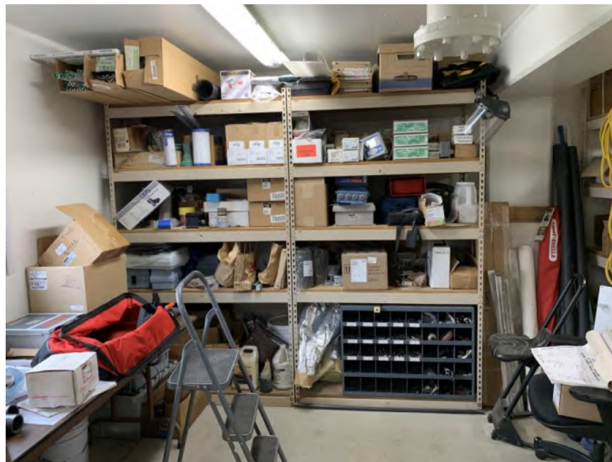
Figure 3.33 – Unrestrained Storage Rack
