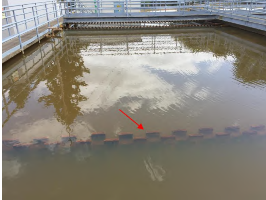
Figure 3.51 – Wooden Baffles in Sedimentation Basin No. 1
