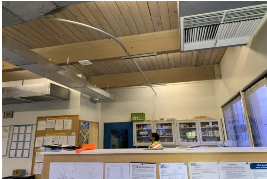
Figure 3.38 – Flexible Diaphragm Chords without Cross Ties
