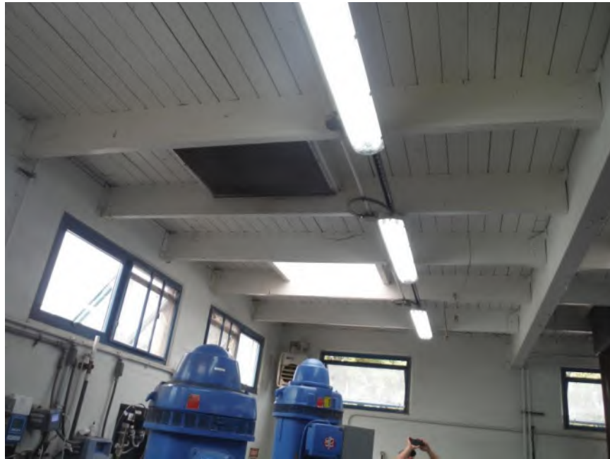
Figure 3.59 – Flexible Diaphragm without Cross Ties
