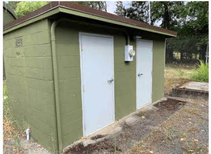
Figure 3.6 – Former Chlorination Building
