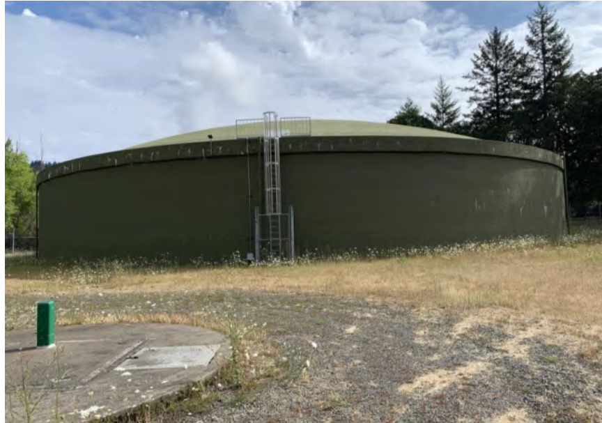
Figure 3.11 – North Valley Reservoir No.2
