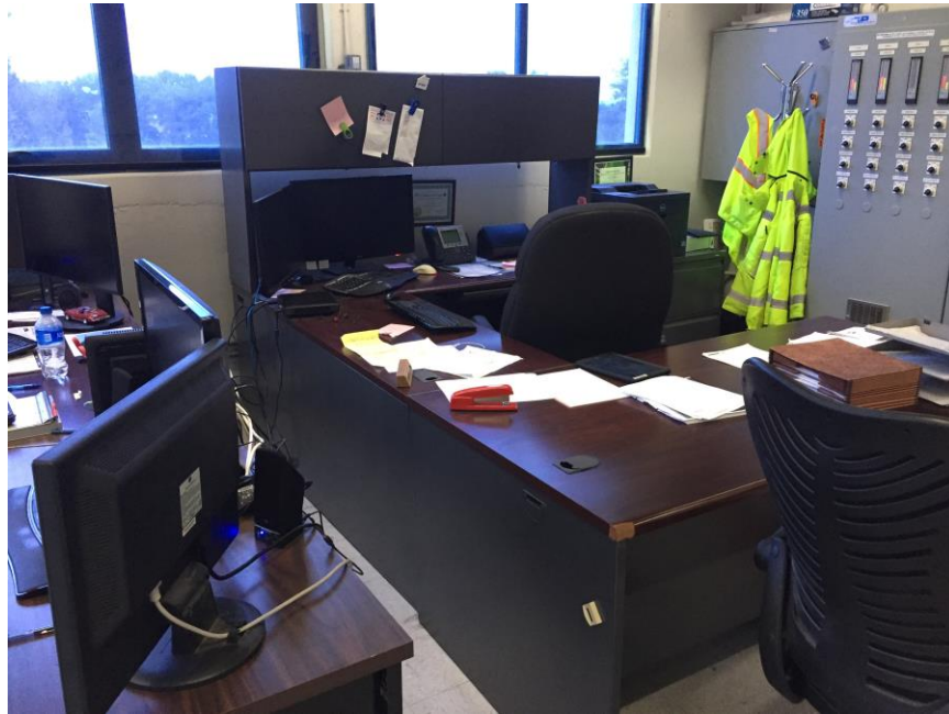
Figure 3.42 – Unrestrained Computer Equipment
