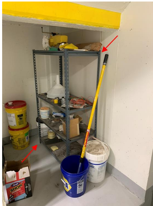
Figure 3.23 – Unrestrained Storage Rack
