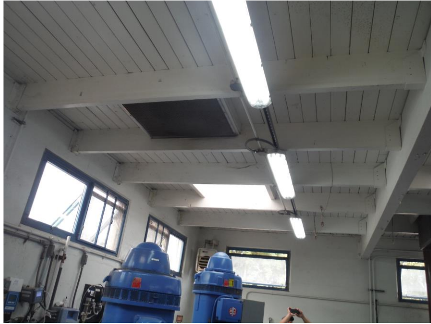
Figure 3.59 – Flexible Diaphragm without Cross Ties
