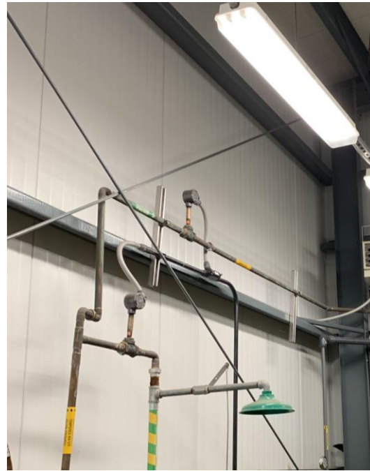
(b) West Bay with Rod Bracing
