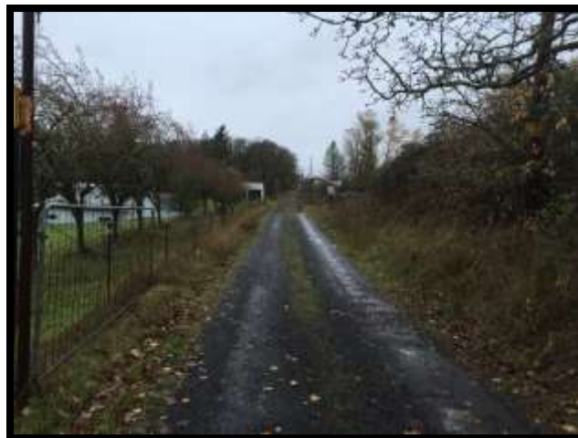
FIGURE 41 NORTH VALLEY RESERVOIR ACCESS ROAD
