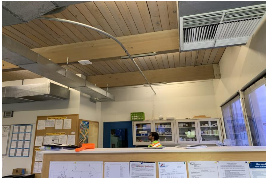
Figure 3.38 – Flexible Diaphragm Chords without Cross Ties
