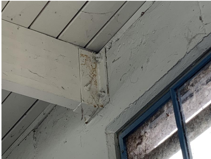
Figure 3.60 – Joist to Perpendicular Wall Connection
