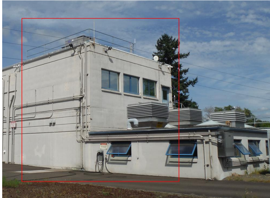
Figure 3.36 – 1970 Treatment/Control Building Addition
