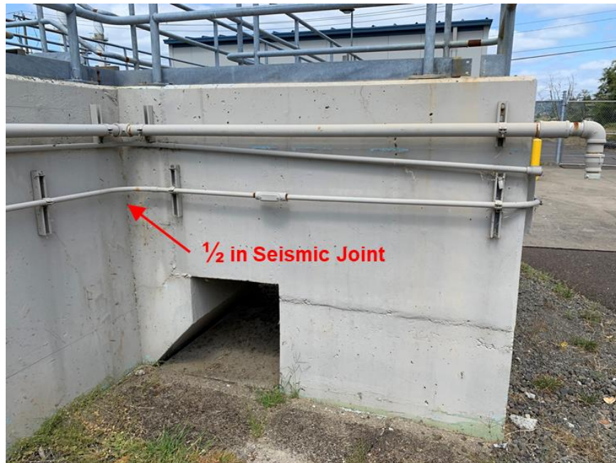
Figure 3.50 – Sedimentation Basins Effluent Structure (Outlet Basin Structure)
