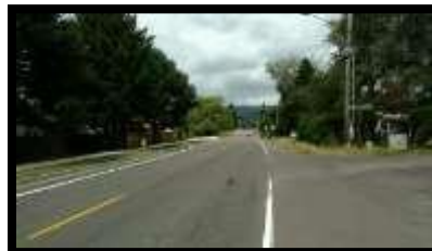
FIGURE 2 LOOKING NORTH ON COLLEGE STREET
