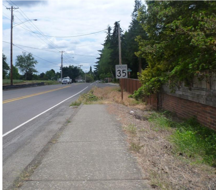
Gaps in Sidewalks on Arterial Roadway
