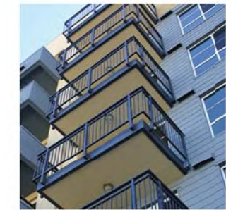
2. ALUMINUM RAILING SYSTEM FINISH: PRE-FINISHED, BLACK ANODIZED
