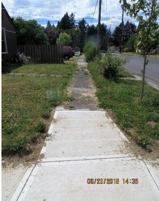
Commonly observed narrow and often disjointed sidewalks with general landscape strip. Photo above shows connection between new and old sidewalk and width difference.
