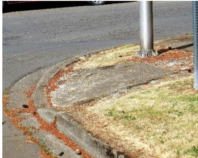
Ramp existence and design varies. In some cases, sidewalks with elevation difference had no existing ramps (right).
