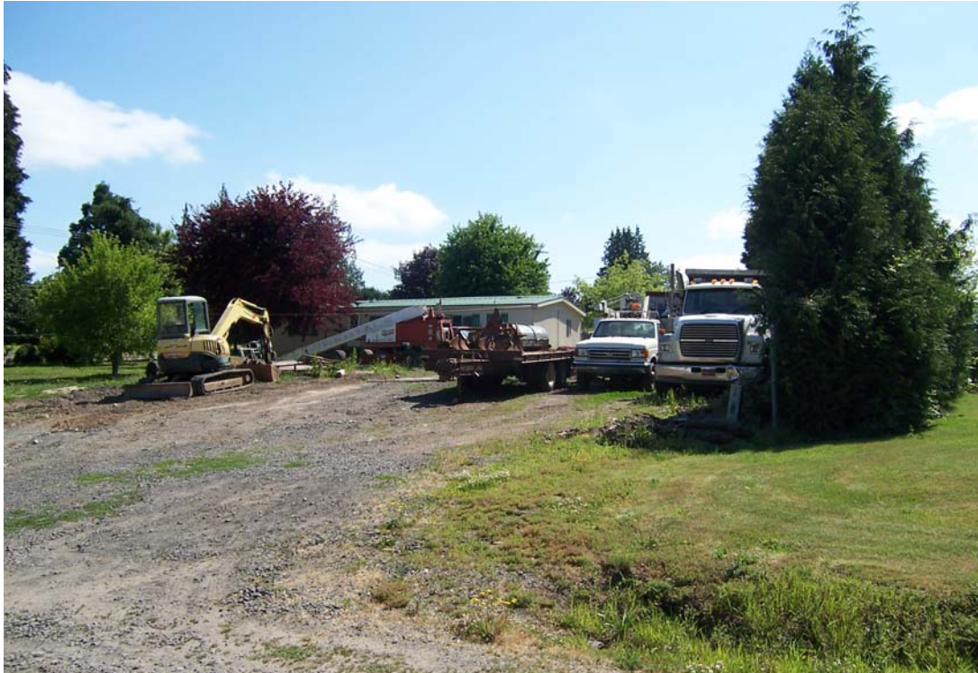
Southwest corner of property
