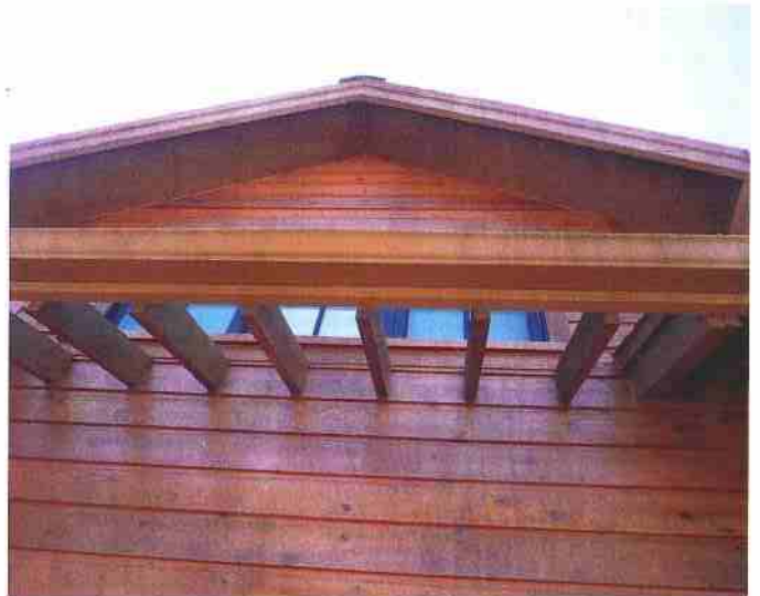
Trellis detail over the current garage door of the residence
