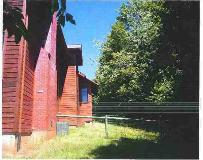
Looking north along the east elevation of the existing building showing proximity of tree line
