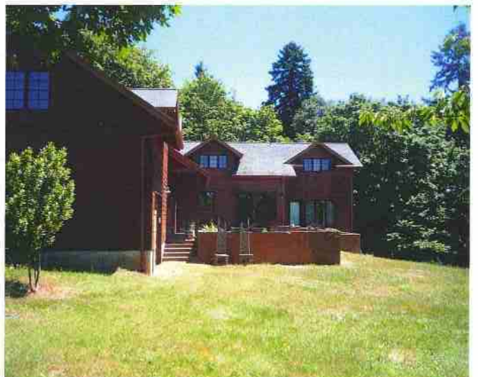
Looking east, showing the existing residence and the future deck area
