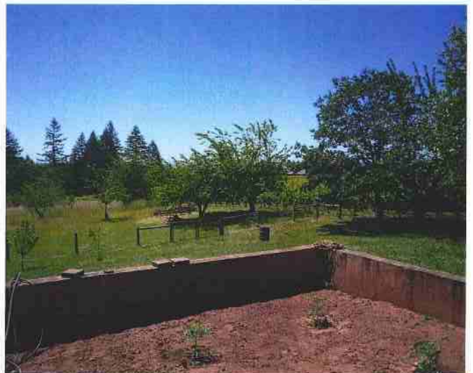
Looking southwest from the future deck area
