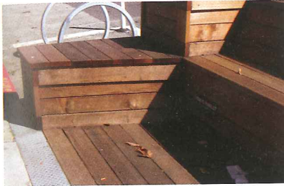
A steel transition plate ensures a flush transition from the curb to the wooden parklet surface.
