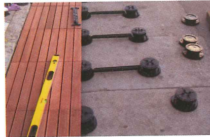
Bison pedestals are a popular substructure for parklets.
