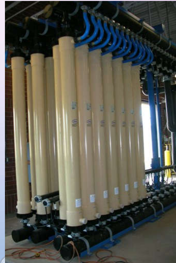
Recycled Water Membrane Filters
