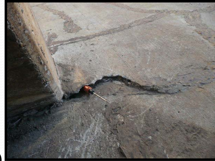
Structural Issues at the Oxidation Ditches
