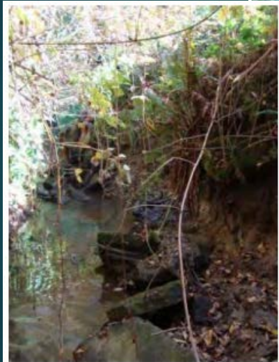
West Bank Chehalem Creek Streambank Erosion
