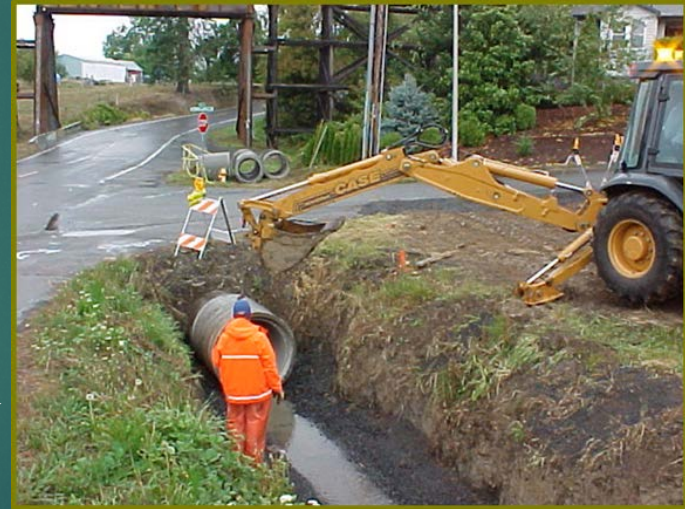
Villa Road Culvert
