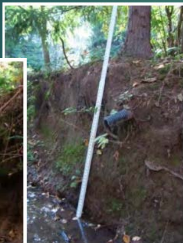
Creek (DS of Mountainview Drive) Residential Stormwater Outfall
