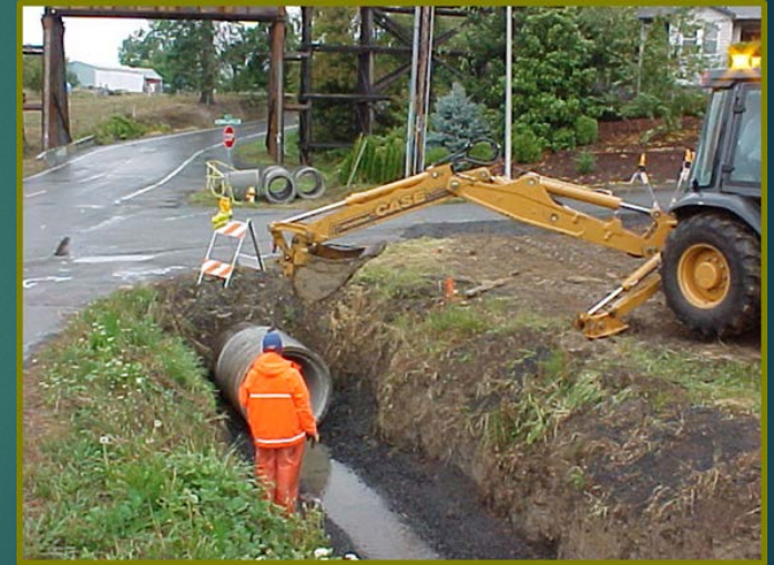
Villa Road Culvert
