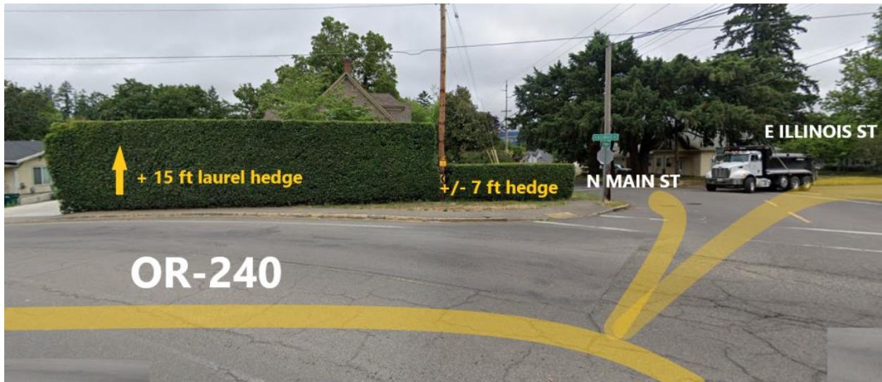
Figure 21. Existing Vegetation and Potential Sight-Distance Considerations at the E. Illinois Street / N. Main Street (OR 240) Intersection. Annotated street-level photograph showing the mature laurel hedges adjacent to the intersection and their potential influence on driver sight distance. Hedge heights shown are approximate and are provided for illustrative purposes only. This exhibit is not intended to represent surveyed conditions, engineering measurements, or a technical sight-distance analysis. A professional sight-distance survey should be conducted to objectively evaluate existing visibility conditions and determine whether vegetation management or other improvements could adequately address identified safety concerns before more intrusive transportation measures are considered.
