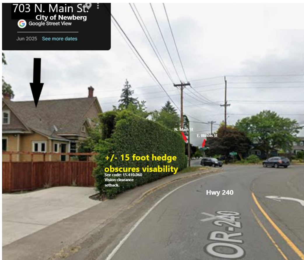
Figure 20. (Author Illustration at left) Existing sight-distance conditions at the E. Illinois Street / N. Main Street (OR 240) intersection. The photograph illustrates the mature laurel hedge that was the subject of Vision Clearance Variance VAR23-0004, approved by the City in January 2024. Approved nearly the same time that the engineering study for the intersection was cancelled.
