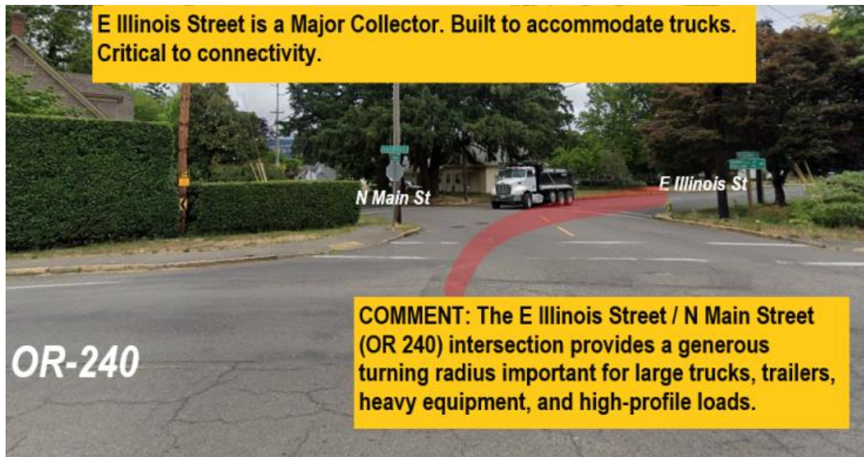
Figure 6. The E. Illinois Street / N. Main Street (OR 240) intersection was designed to accommodate the turning movements of trucks, commercial vehicles, trailers, heavy equipment, and oversized loads traveling between OR 219 and OR 240. The generous turning radius reflects the corridor's long-established function as a Major Collector serving industrial properties, freight movement, and regional connectivity.
