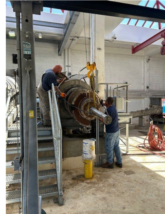
Installing repaired screw
